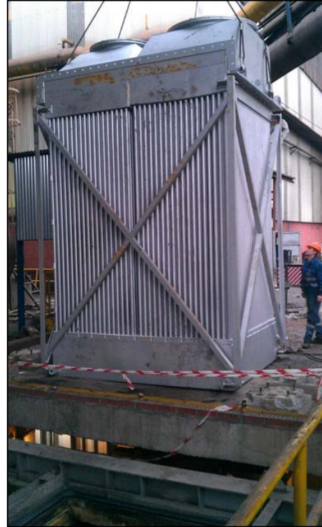
b) New recuperator assembly
