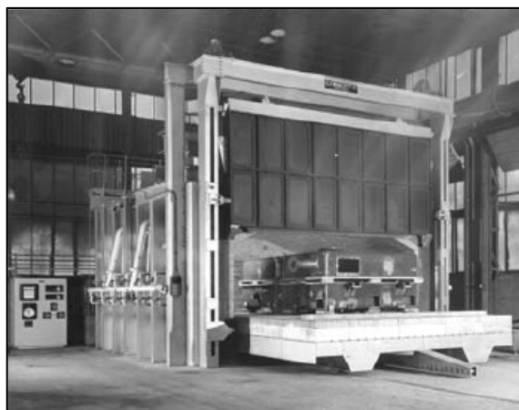
Figure 3.3. Two large gearbox cases entering a large annealing furnace [29].
