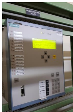
Figure 3.14. Distance relay.
