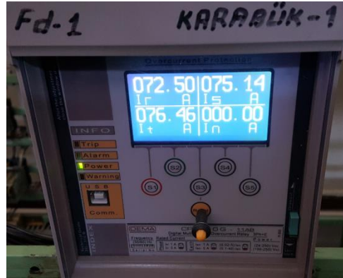
Figure 3.9. Overcurrent relay.
