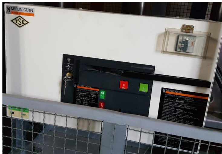
Figure 3.3. SF 6 gas circuit breaker.
