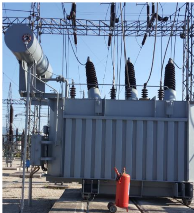
Figure 3.4. Power transformer.
