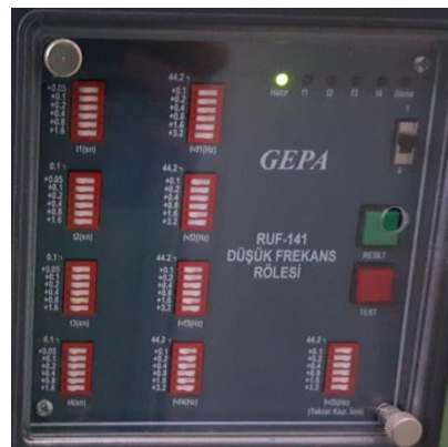
Figure 3.15. Frequency protection relay.
