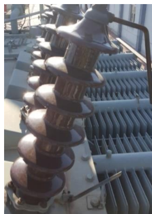
Figure 3.7. Spark gap.
