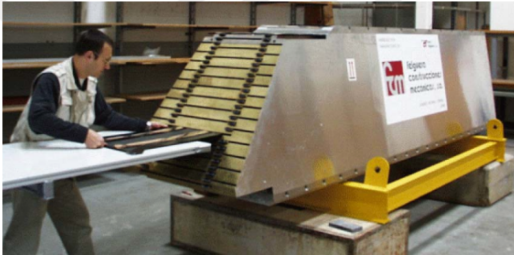
Figure 2.12: Installation of a central megatile.
