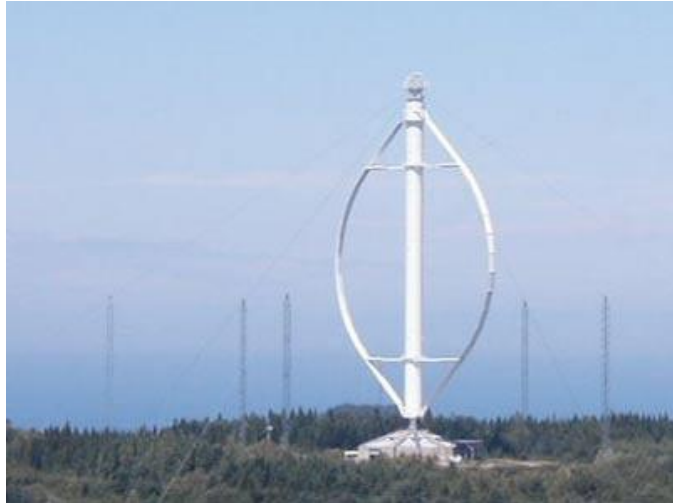
Figure 2.3. Darrieus VAWT (Deisadze et al. 2013).
