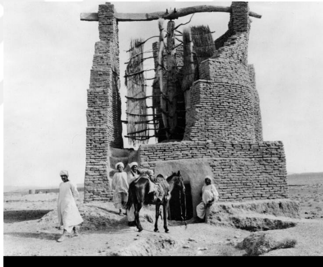
Figure 2.1. Vertical-axis windmill for milling grain, Afghanistan (Hau, 2006).
