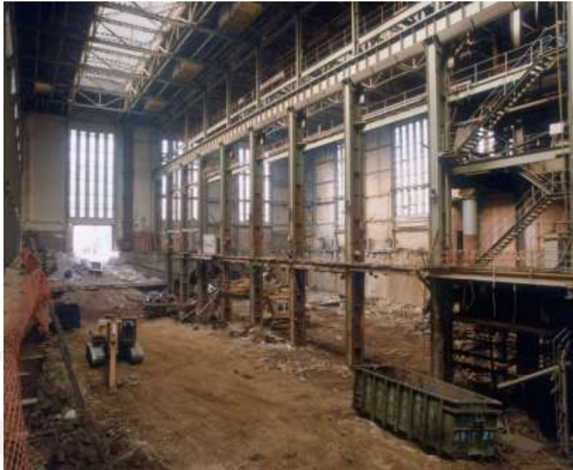
Figure 4.6 Bankside Interior – Photo © Marcus Leith, Tate - Source: Tate Modern Web Site
