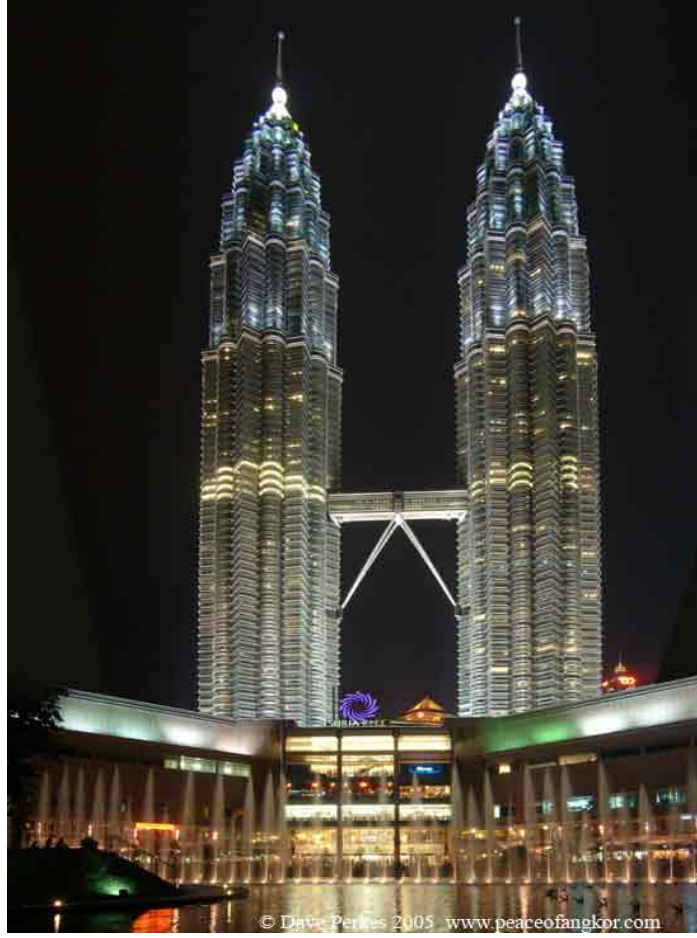
Resim1-2: Petronas Towers ( Kuala Lumpur )
