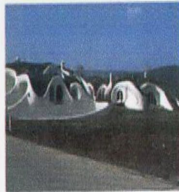
Nine Houses, Peter Vetsch
