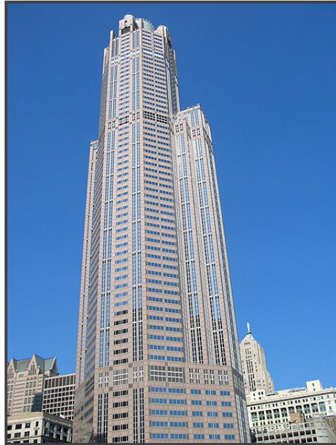
Şekil 3.19 : 311 South Wacker Drive
