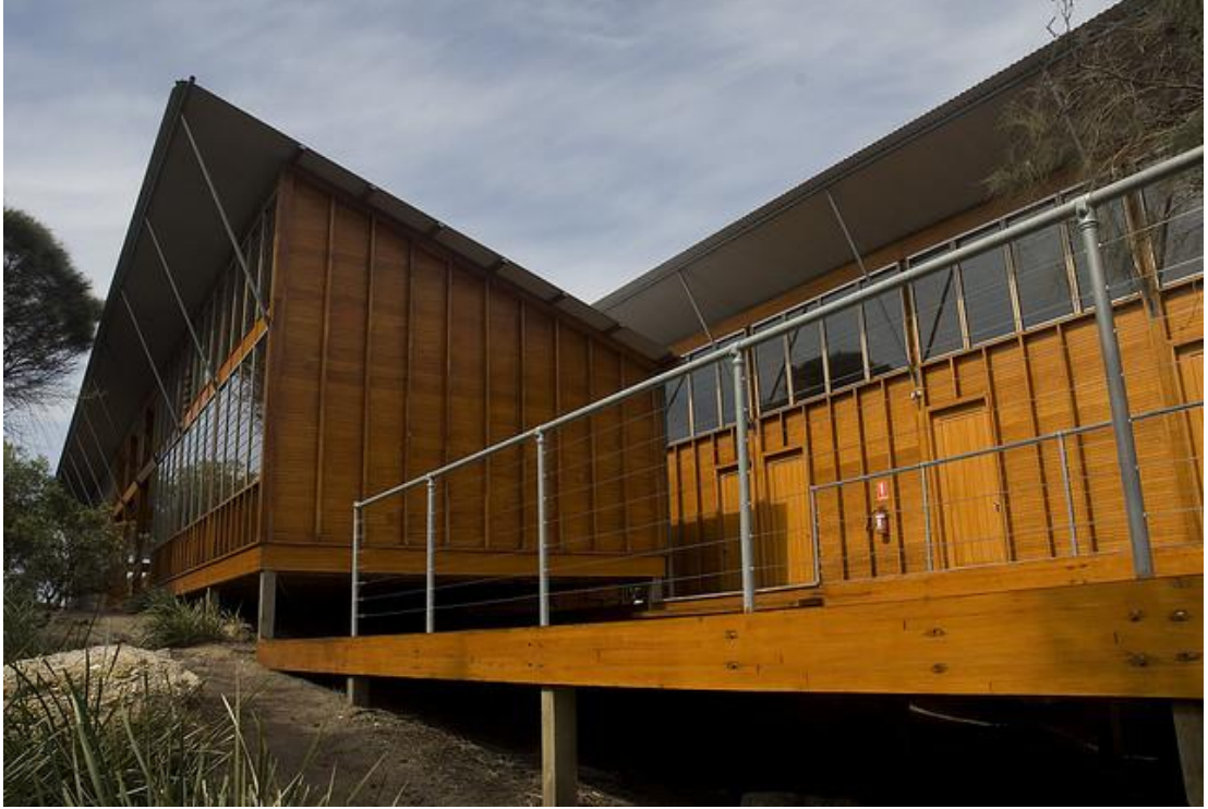
Şekil 61. “Bay of Fires Lodge” Otel URL-61: https://encrypted-tbn3.gstatic.com/images
