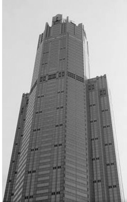
Şekil 2.4 - South Wacker Drive
