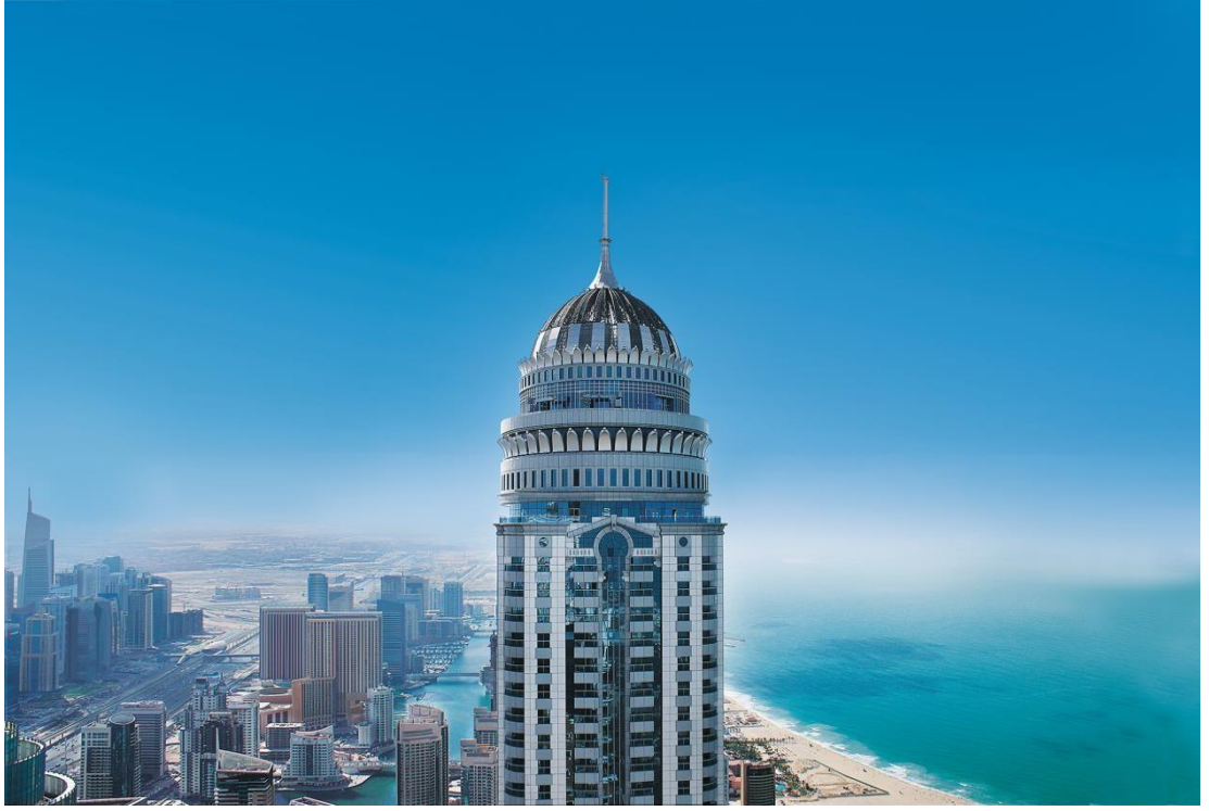
Şekil 2.42. Princess Tower (URL – 57)
