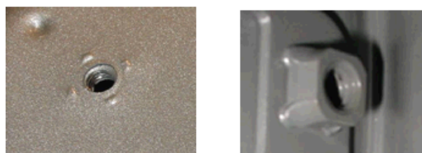
Figure 4.5 Weld Nut Connection
