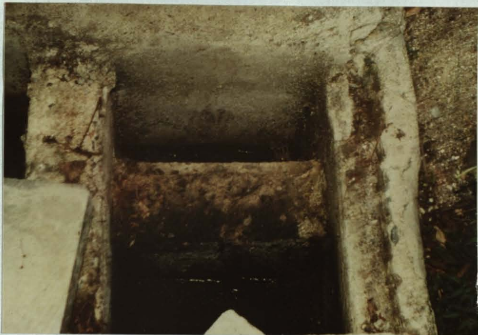
Figure 11 : Photograph of the Concrete Wall at the end of the Channel
