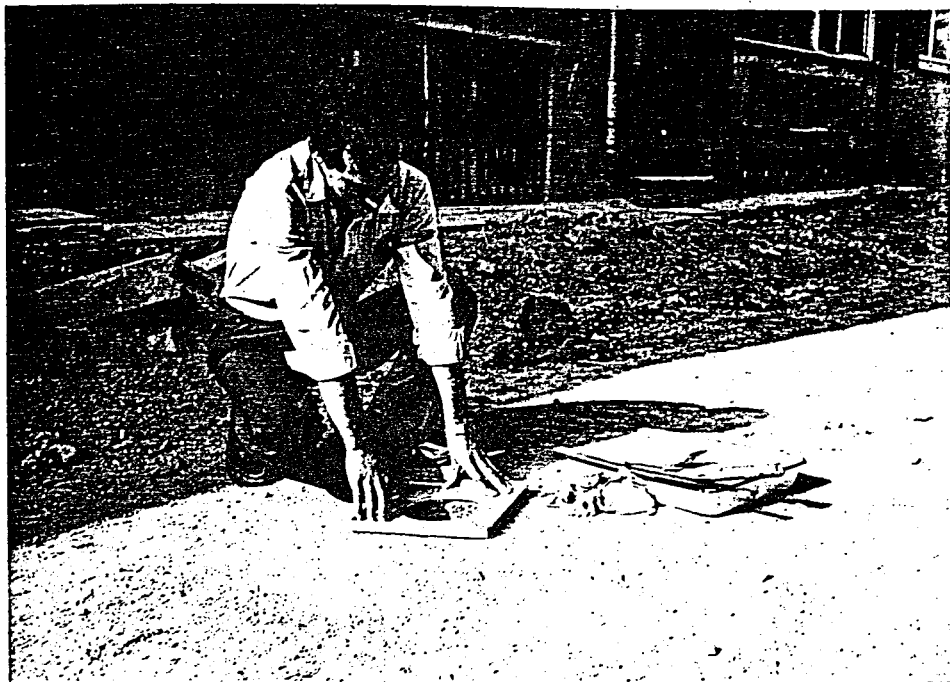
Figure 2.3 _ FIELD DENSITY TEST _ BASE PLATE PLACEMENT AT KADIKÖY YELDEĞİRMENİ REGION
