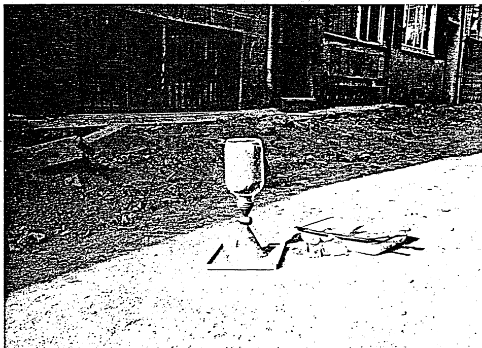
Figure 2.4 _ FIELD DENSITY TEST WITH SAND CONE APPARATUS AT KADIKÖY YELDEĞİRMENİ REGION
