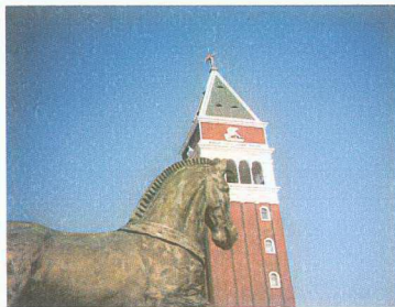
Figure 4-20 The Campanile Tower , VPRH.
