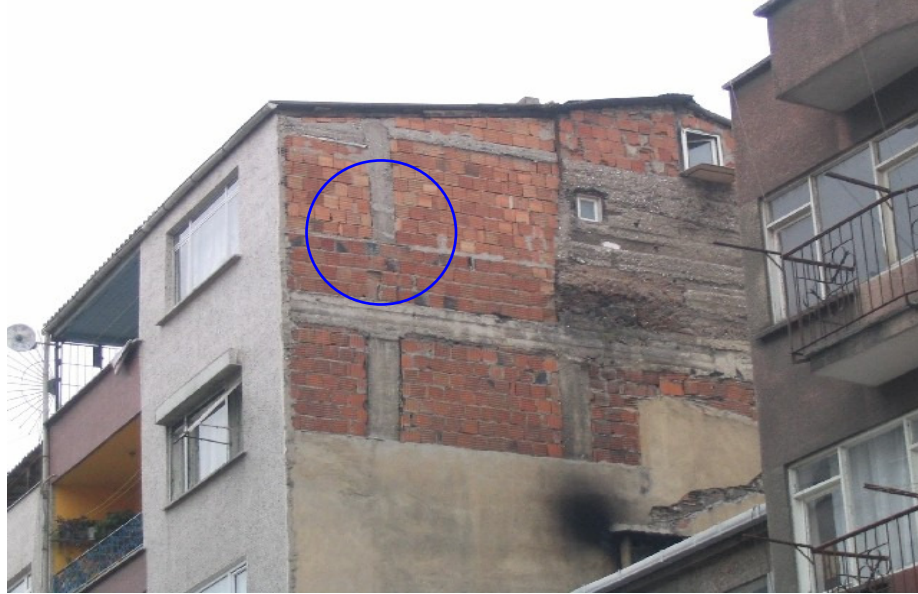
Figure 2.1. A building in İstanbul that has discontinuity in one of its columns
