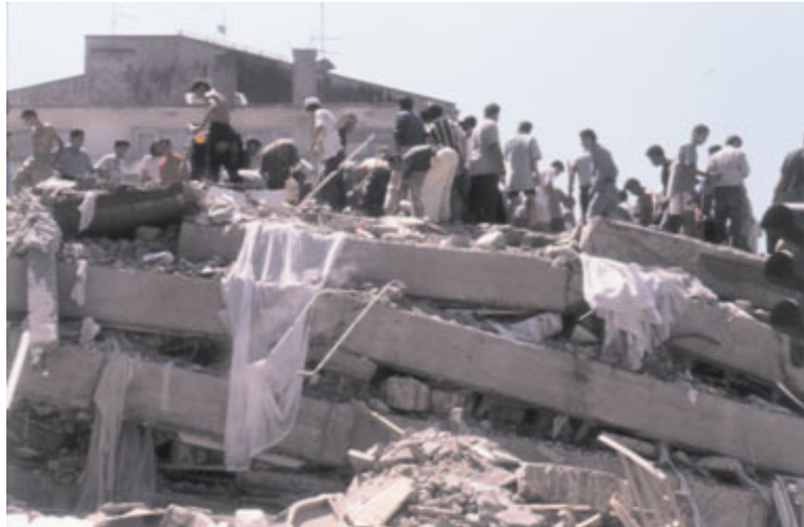
Figure 1.6. A completely destroyed building.
