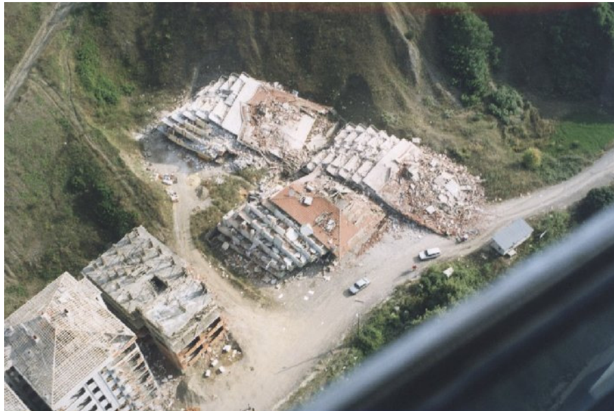
Figure 2.4. Buildings that are completely collapsed during an earthquake.
