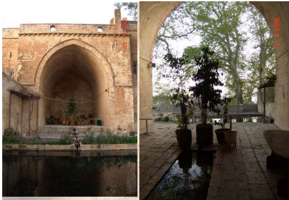
Picture 4.2.13 Water Channels in Interiors (Kasimiye Medresseh)
