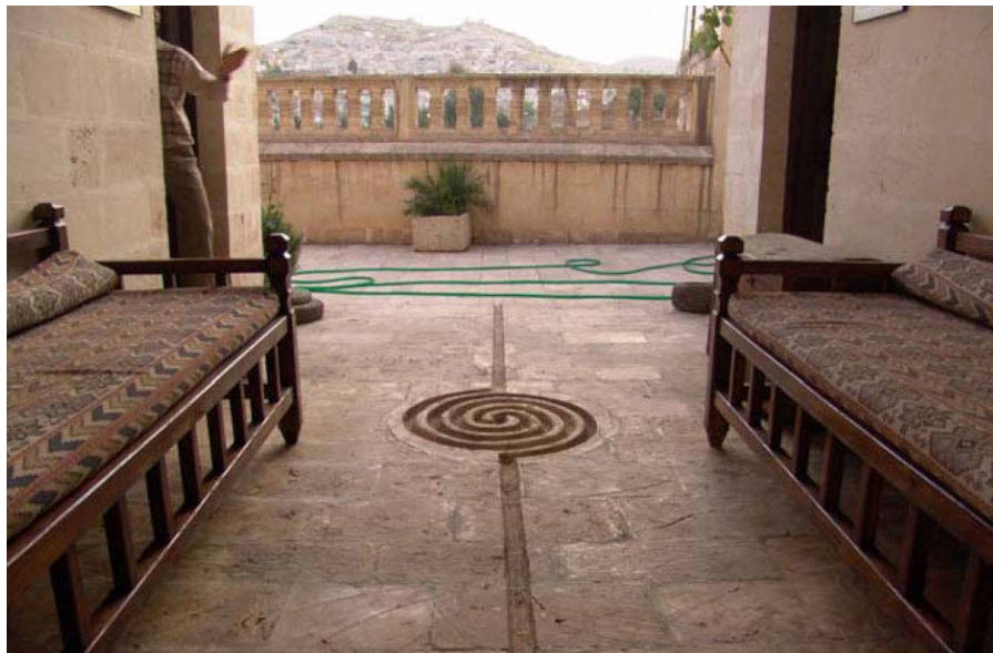
Picture 4.2.11 Water Channels on The Ground (Mungan House)
