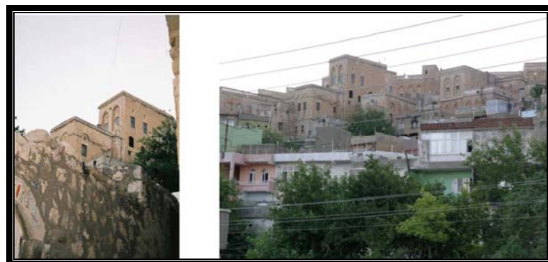
Picture 4.1.5 Mungan House
