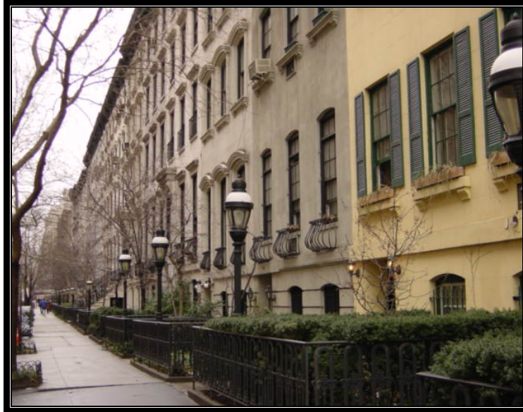
Picture: 2.1.2 A London Terrace had Wooden Shutters
