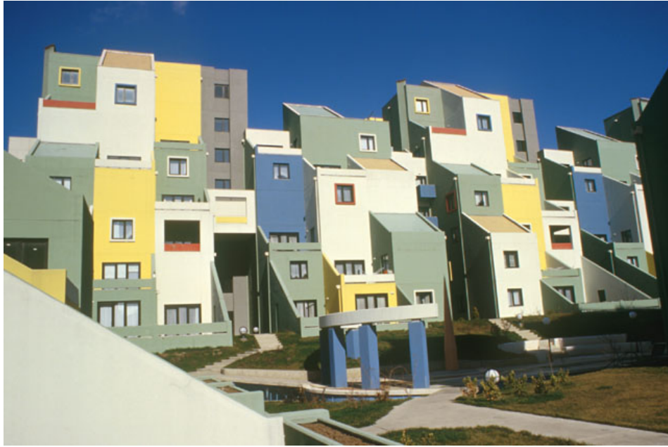
Picture 4.1.1 Contemporary Architectural Sample of Daylight Gain (Sürücüler sitesi Ankara –Melih Karaaslan)
