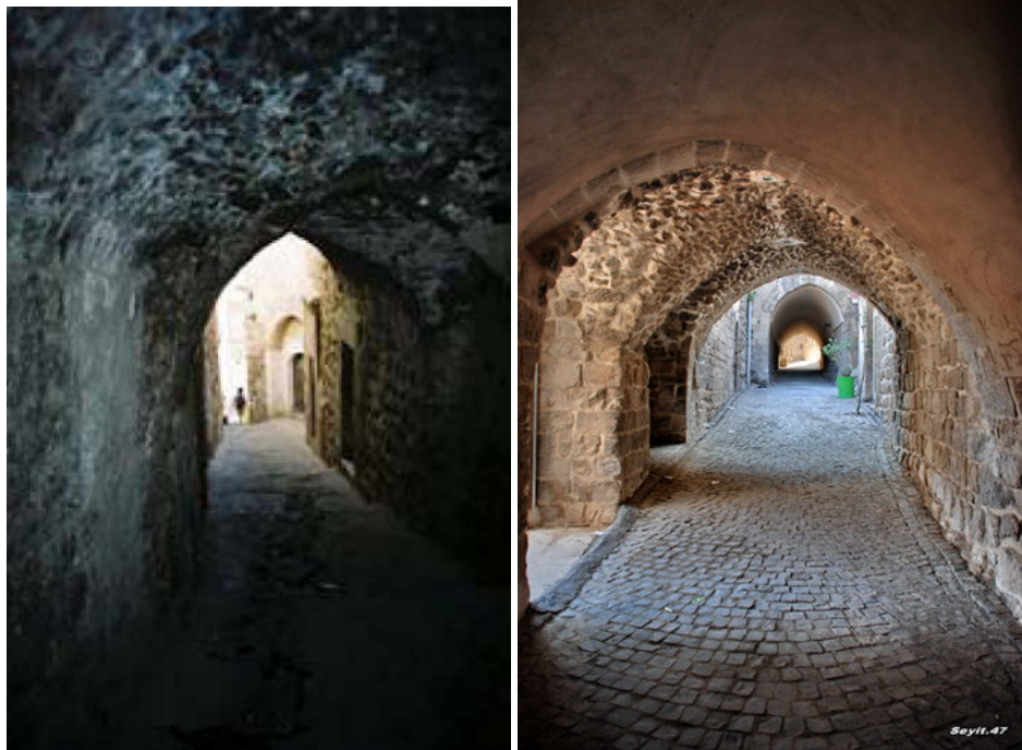
Picture 3.2.5 Creating Shade Space in Hot Summers Photo: Nilay Ünsal Gülmez from Bazaar in city center.
