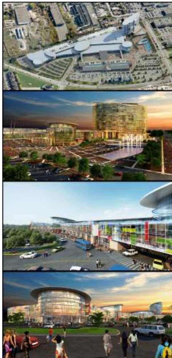
Figure 2.5. Remington Centre, north of Toronto, will have a vast outdoor public space (Canada's largest multi-cultural shopping center's ground breaking is expected in 2011) ( http://www.worldarchitecturenews.com/index.php?fuseaction=wanappln.projectview&upload_id=13055(22.12.2009) )
