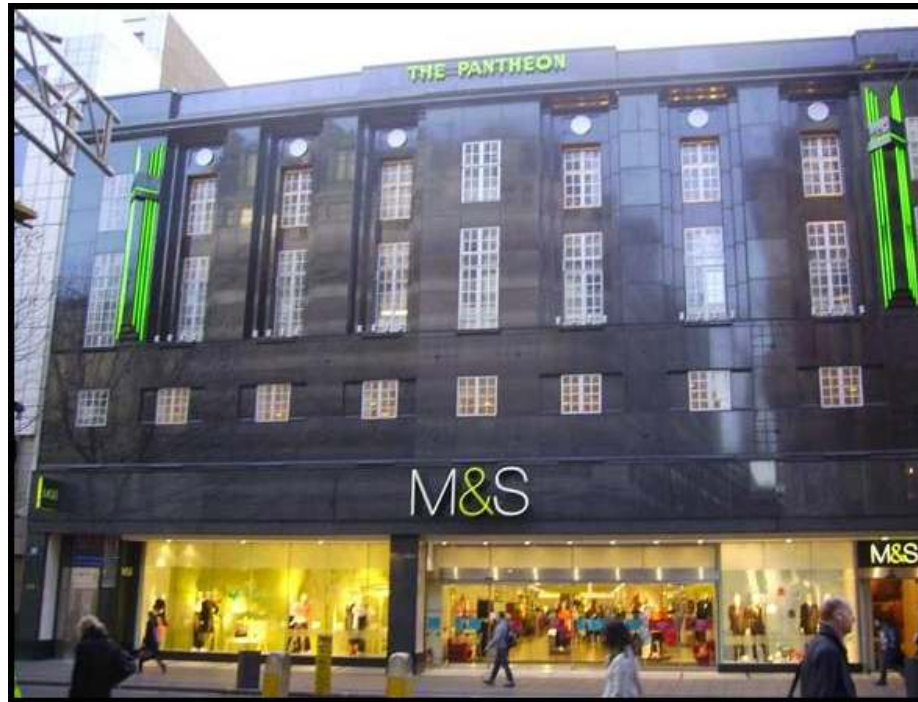
Figure 3.20. Marks and Spencer's 'Oxford Street Pantheon' branch ( http://www.macegroup.com/projects/project-library/marks-and-spencer-pantheon-store (12.12.2009))
