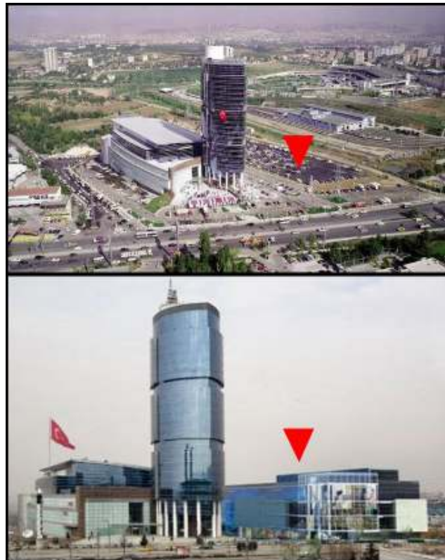
Figure 5.2. Armada Shopping Center and future expansion (under construction currently)
