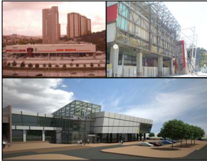
Figure 5.3. Mesa Plaza shopping mall, Ankara One of the oldest shopping malls in Ankara is having an overall renovation. ( http://mw2.google.com/mw-panoramio/photos/medium/16373606.jpg (12.12.2009)) ( http://img193.imageshack.us/img193/4323/dsc01267g.jpg (12.12.2009)) ( http://www.mardav.com/HaberResimler/48744067cam-01-0002 .jpg (12.12.2009))
