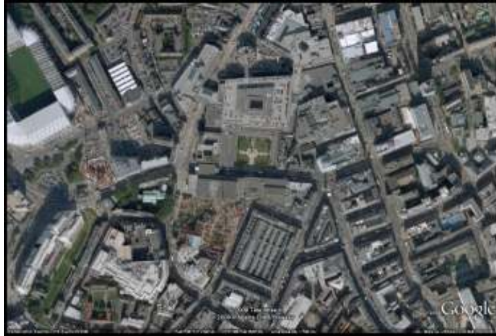
Figure 4.24. Eldon Square Shopping Centre (Google Earth (12.12.2009))
