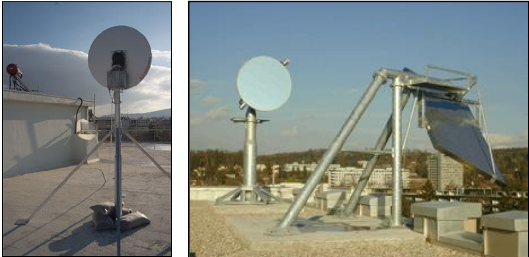
Figure 3.7 Heliostat Appropriately Located and Oriented to Provide Sunlight on The Requested Surface
