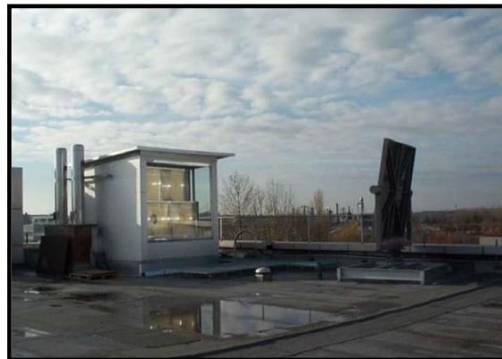
Figure 3.10 The Heliostat on Top of The Semperlux Building in Berlin, Germany.
