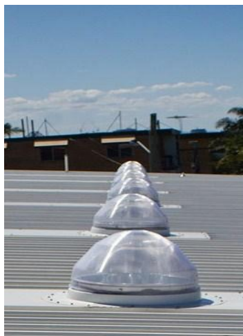
Figure 3.11 Sunlight Tracker of Mirrored Light Pipes in The Roof.
