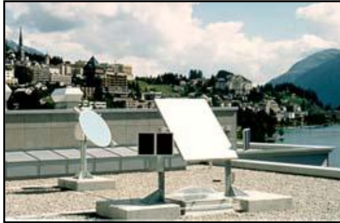
Figure 3.8 White Hologram Appropriately orientated at the suitable inclination in accordance with its optical properties deflects sunlight so that it flows vertically into the narrow light shaft reaching even the last windows
