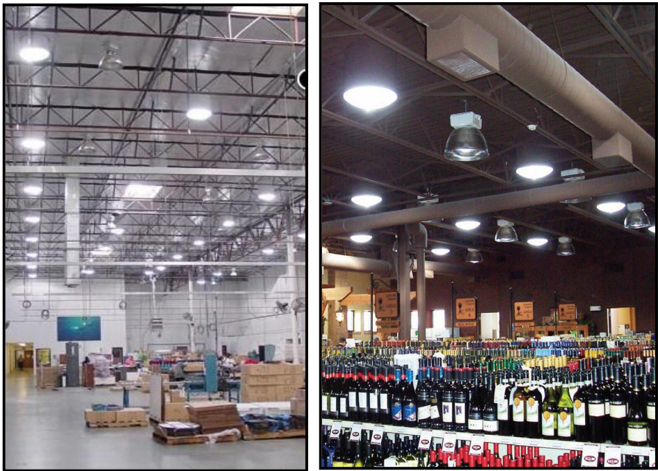
Figure 3.13 Mirrored Light Pipes Use in Supermarket-South London
