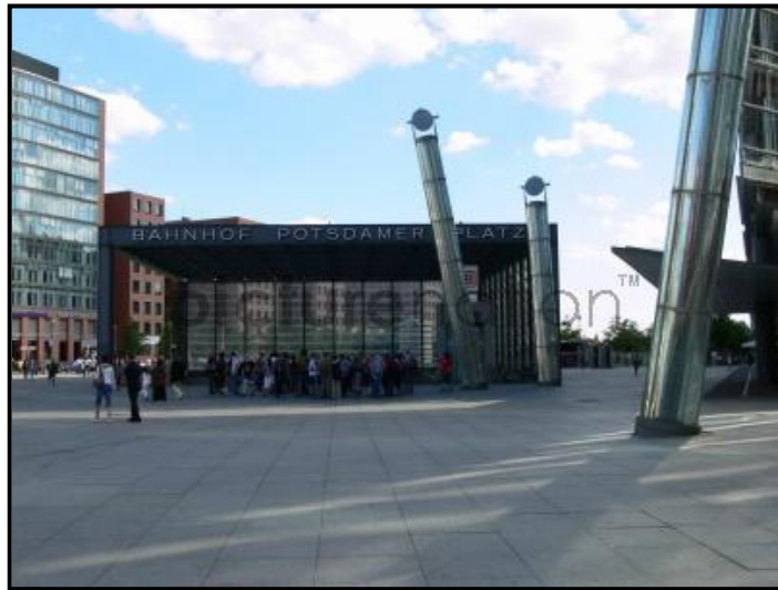
Figure 3.23 Light Pipes, Subterranean Train Station at Potsdamer Platz, Berlin
