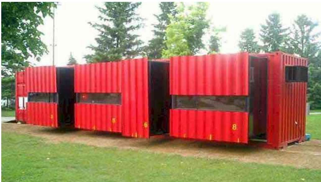
Figure 17. The First example of container house, built by Mark Podlaseck and hispartner, Steve Bryant. Name is MDU House. [83]
