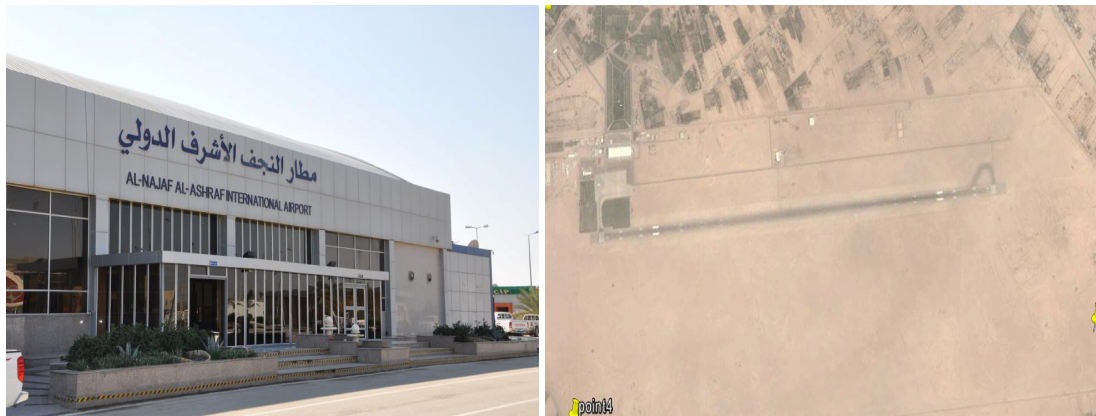
Figure 14 Al-Najaf International Airport
