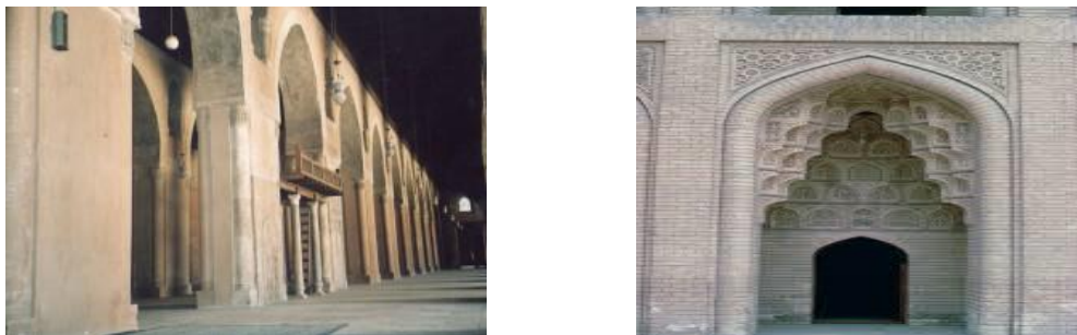
Figure 7: Pillar & pointed arch & Abbasied Palace Baghdad_ foil arch.
