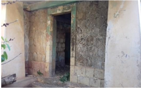
Figure 64. Shows the front entrance of the house and of the Italian-style
