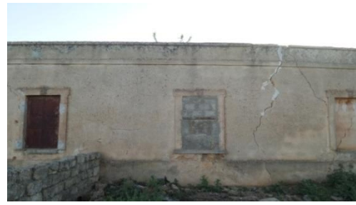
Figure 58. Showing the right side of the house and the windows cracked in the presence of the wall and not fit for habitation
