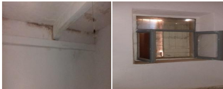
Figure 55. Shows the window and the roof from the inside without a change in the Italian style
