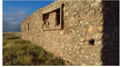
Figure 79. Showing the left side of the house
