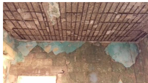
Figure 69. Showing the house roof and show the materials used
