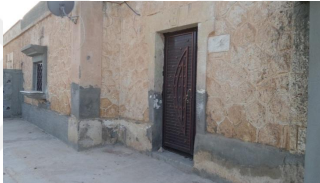
Figure 25. The front of the house shows the change only in the door
