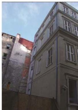
Fire escape windows have been opened. Entire of the rear wing facade has been uncovered after demolition of adjacent buildings.
