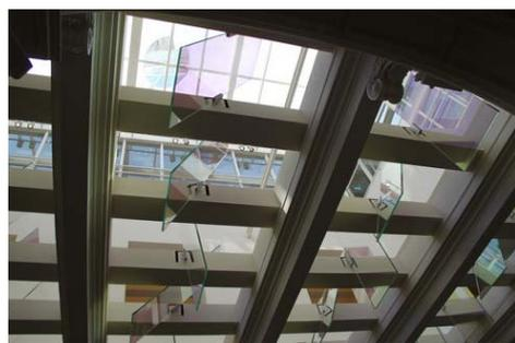
**Figure 3.59** Salt Galata's mirror panels (heliostats)
