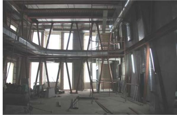
**Figure 5.13** Elevator structure was installed while construction of 2<sup>nd</sup> and 3<sup>rd</sup> floor gallery void was still ongoing (GAD, November 2008)
