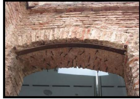
**Figure 3.19** Belt reinforcement
