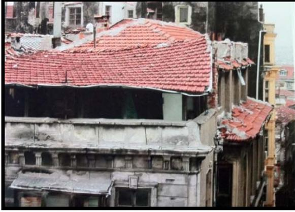
**Figure 4.35** Marseille roofing tile has been used in roof. The roof is in the form of hipped roof
