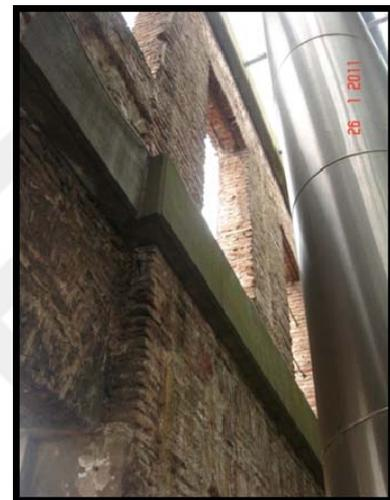
**Figure 3.20** Retrofit reinforced concrete brace or wrapping
