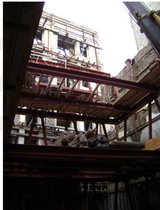
**Figure 5.3** Diagonal structure is being erected as the steel beams are placed between the layers (GAD, March 2008)
