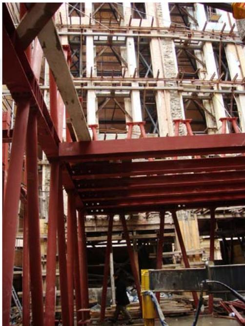
**Figure 5.2** Steel supports are used to keep the frontal facade standing (GAD, February 2008)
