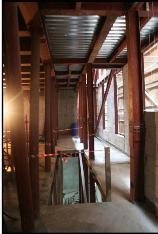
**Figure 4.59** Diagonal steel structure is seen on the left side, I steel columns are seen on right side, gas concrete blocks are seen on right front, steel right profiles used in horizontal are seen at the top
