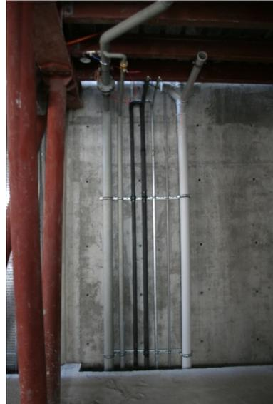
**Figure 5.11** Electricity and installation pipes were installed in the shafts (GAD, September 2008)
