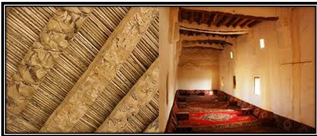
Figure 64 Roof of An House in Village Built By Mud and Roff by Palm Trankes, (Researcher).
