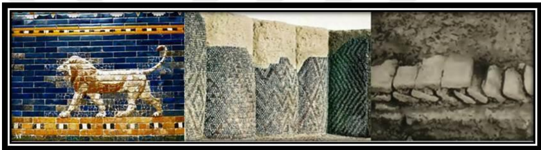
Figure 17 Glazed Brick (Ishtar Gate) [59] , Glazed Brick in Kish Palace Hall Covered Wall And Columns [65], and Backed Brick Built in Decorative Way, [65].
