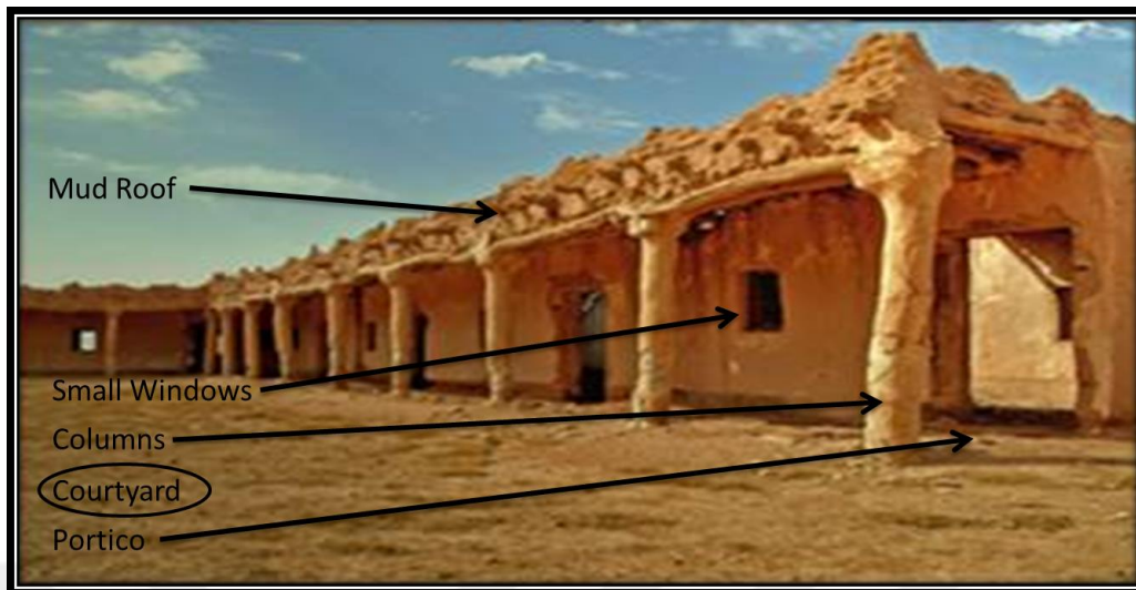
Figure 65 Old Big Mud House, Appear in Picture, Size of Windows, Portico, L shape Plan, and Courtyard, in Diyala, Iraq, (Researcher).
