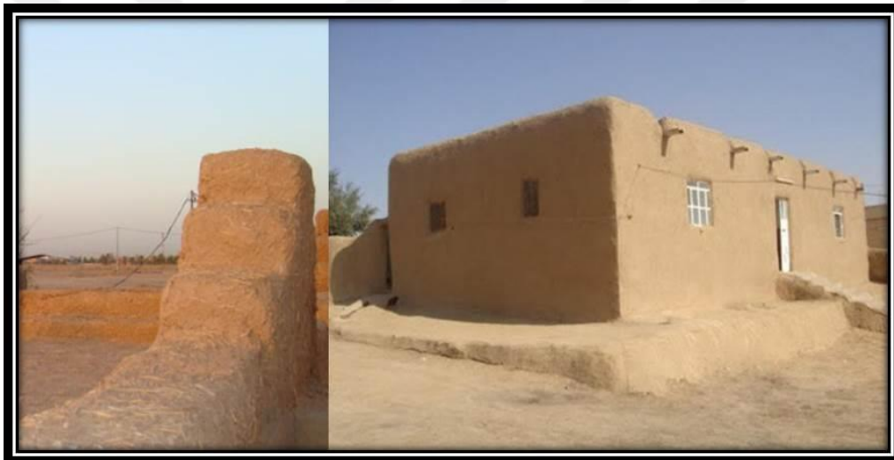
Figure 63 “Ttof” Way of Built in Addition to Mud Brick, and Mahdef in House of Mud in Village in Diyala, Iraq, (Researcher).
