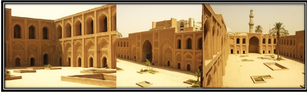
Figure 22 Al-Mustansiriya School, Baghdad, built in Abbasside Period [141], [3], [3].
