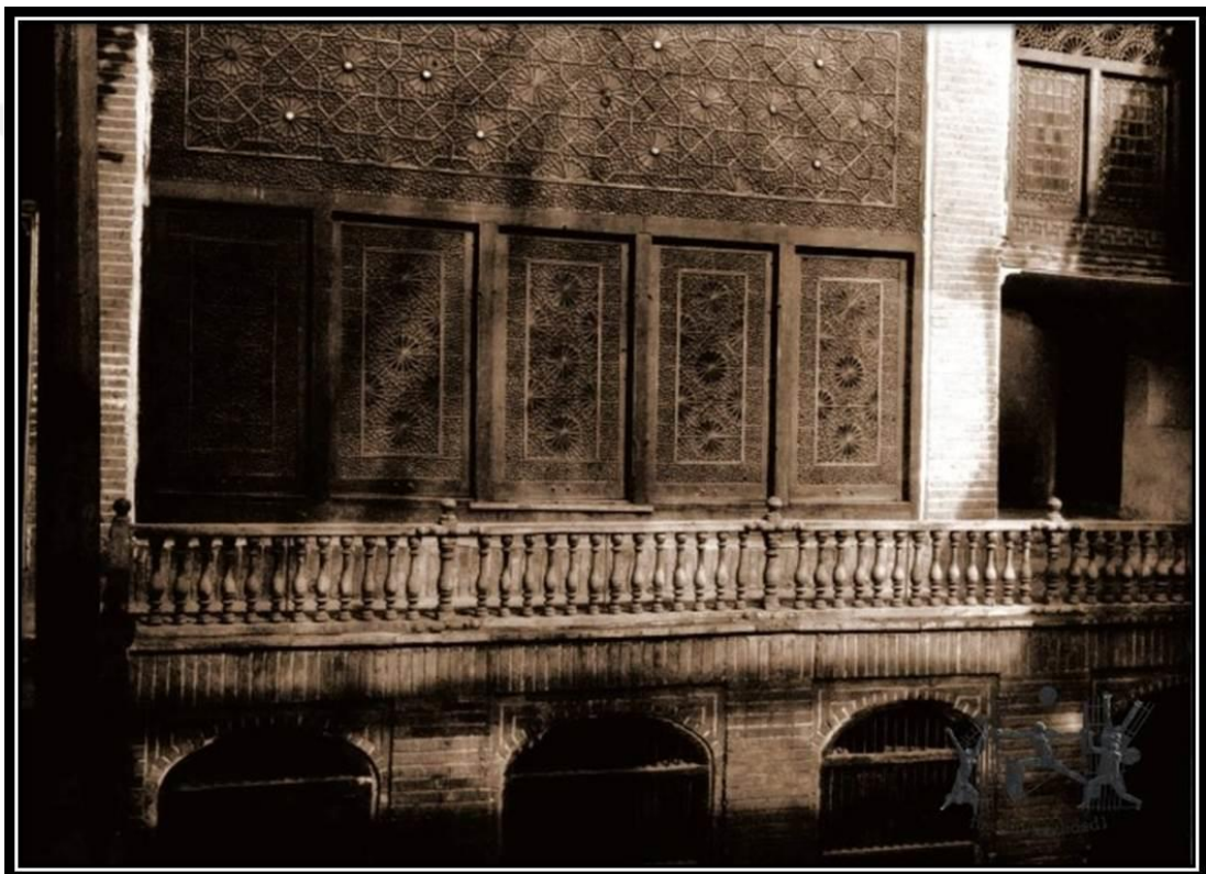
Figure 69 Ursi in Traditional Iraqi Houses, Facing Courtyard, in Addition Portico Appear with Talar in Ground Floor [112].
