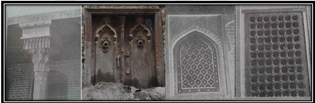
Figure 74 Wooden Head of Column in Shashor House in Baghdad [152], Ornamented Wooden Gate in Baghdad[145], and Grill Windows in Manahim House in Hillah [152].
