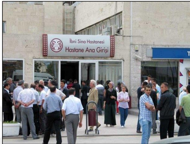
Figure 4.6. The main entrance of İbni-Sina Hospital
