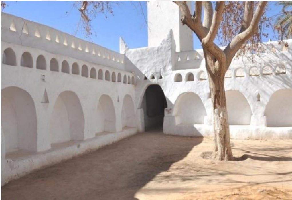
Figure 3.12: The same square of Figure 3.10 after restoration works(GDA, 2007)
