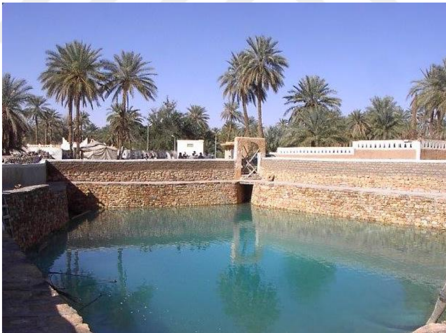
Figure 3.8: Ain Al Faras, the main water source and the center of the old city of Ghadames, after restoration works(GDA, 2007)
