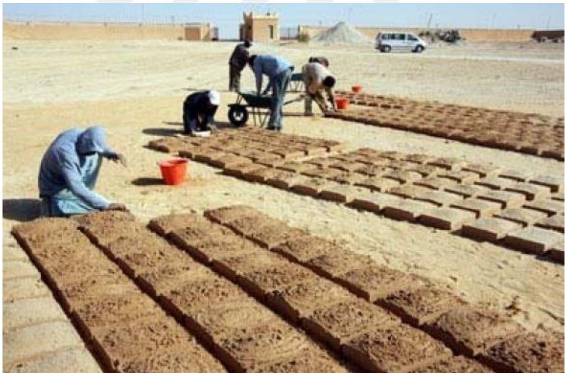
Figure 3.30: Adobe bricks production as part of the restoration works (Auroville Earth Institute, n.d.)
