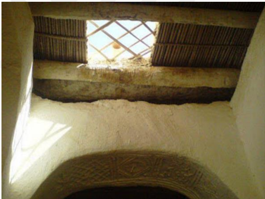
Figure 3.17: Natural lighting and ventilation openings at the roofs of the streets (Tinnaot) (Fteita, 2012)
