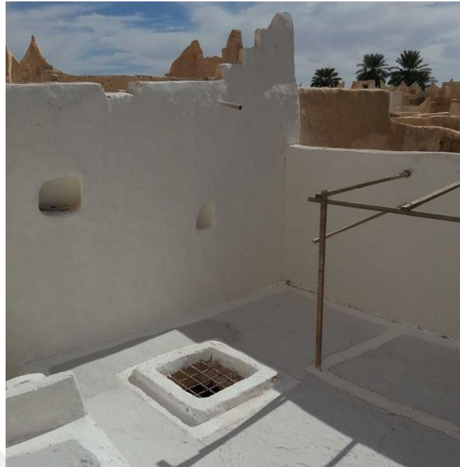
Figure 3.28: Wall and ceiling openings (Tinavot) in traditional houses (Elwefati, 2007)
