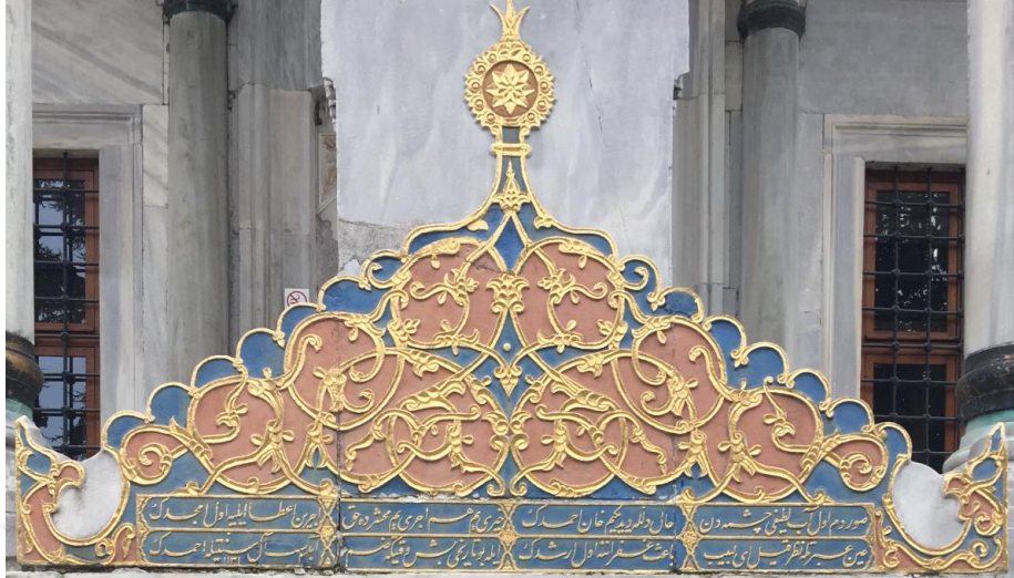
Figure A6: Topkapi Palace - Sultan Ahmed I library fountain - Fountain decoration - Marble engraving and painting
