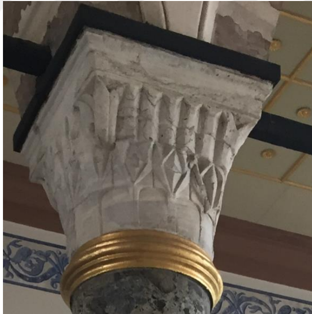
Figure A4: Topkapi Palace - Sultan Meeting room - Column Head - Marble engraving with Golden and marble accents
