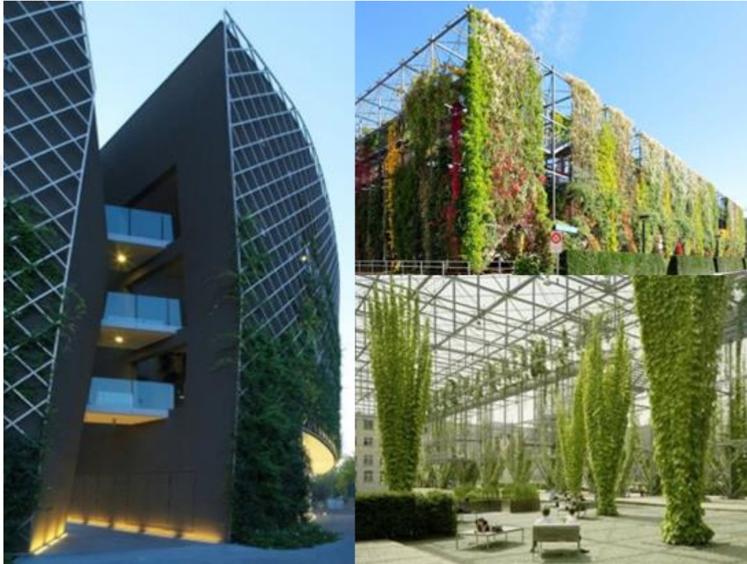
Figure 2.15: Examples of the grid system (left picture) and wire and rope systems (right pictures) (Timur & Karaca, 2013, p. 591)
