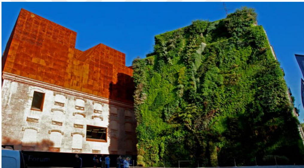
Figure 2.16: Mat living walls example from Spain (Timur & Karaca, 2013)
