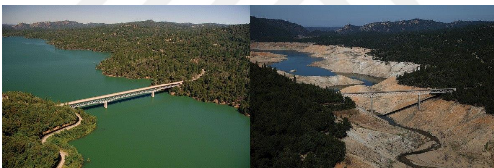
Figure 2. 23: The Enterprise Bridge passes over a section of Lake Oroville in 2011 (left) and 2014 (right) in Oroville, California, which is experiencing “exceptional” drought.” (Sevett, 2015)
