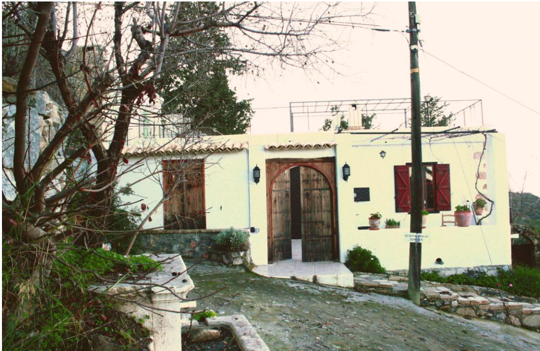
Figure 4. 1 Example of a vernacular house in Northern Cyprus (Movahedi, 2012).
