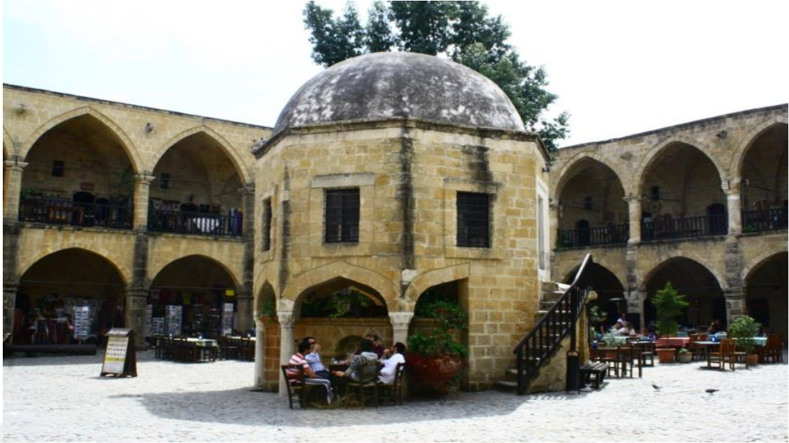
Figure 4. 13 Water source in yard of a vernacular public building (Movahedi, 2012)
