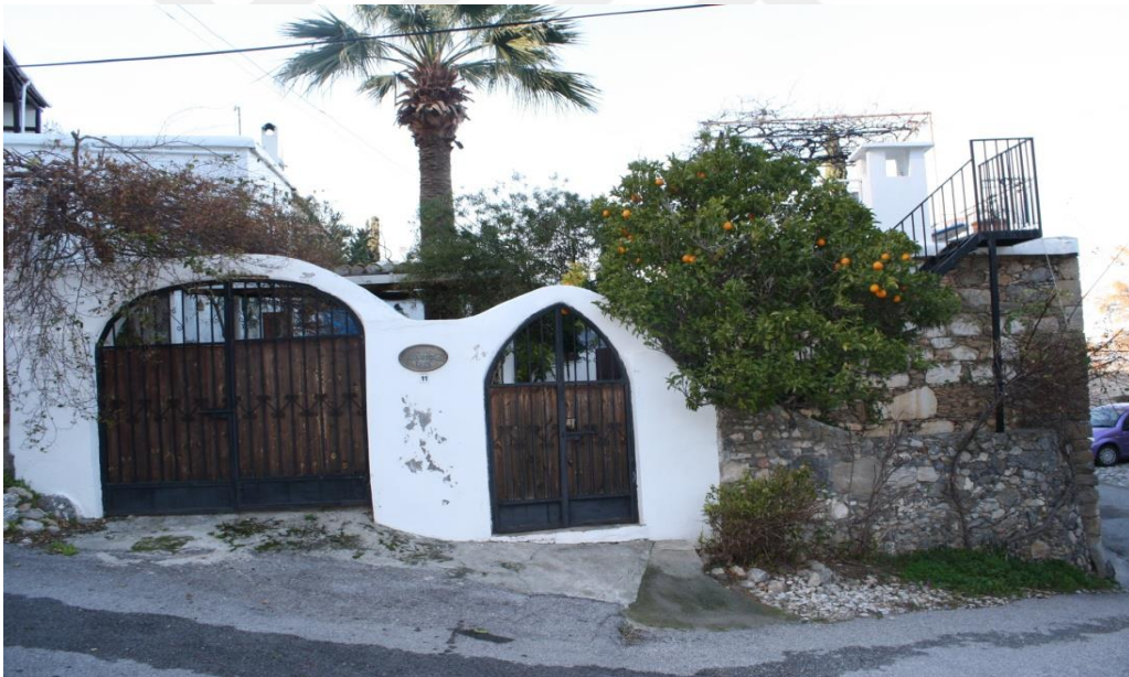
Figure 5. 12 South side wall and entrance of House 1 (Movahedi, 2014).
