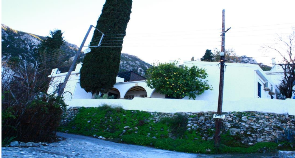
Figure 5. 15 Exterior Walls of House 2 (Movahedi, 2014)
