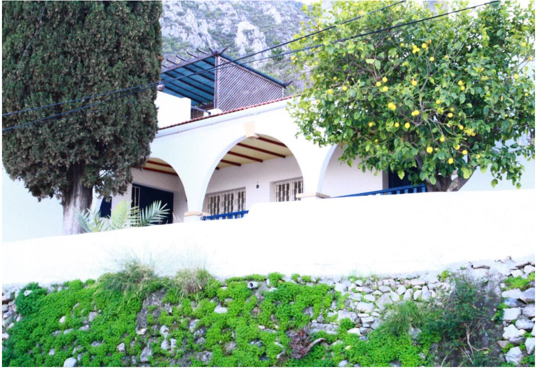
Figure 5. 17 North side-walls second example (Movahedi, 2014)
