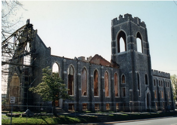
Figure 15. Image of the church before reuse (Source: FMK architects, 2002)
