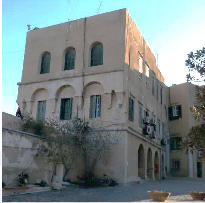
Figure 4.7: A building in Tripoli Castle where modern utilities have been added without a clear rehabilitation plan, ruining its historical and cultural values. (Author's collection)
