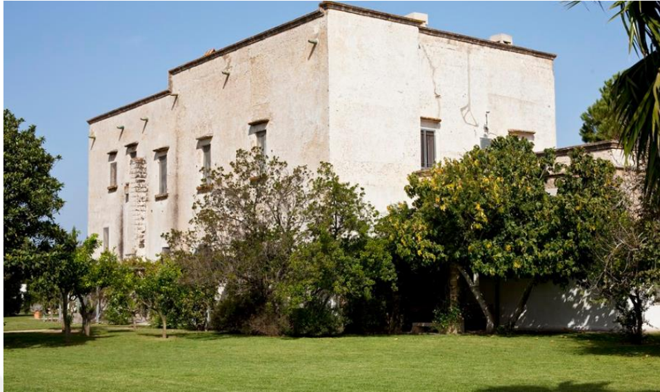
Figure 3.2: Exterior of Villa Elia (The Thinker Traveller, 2018)
