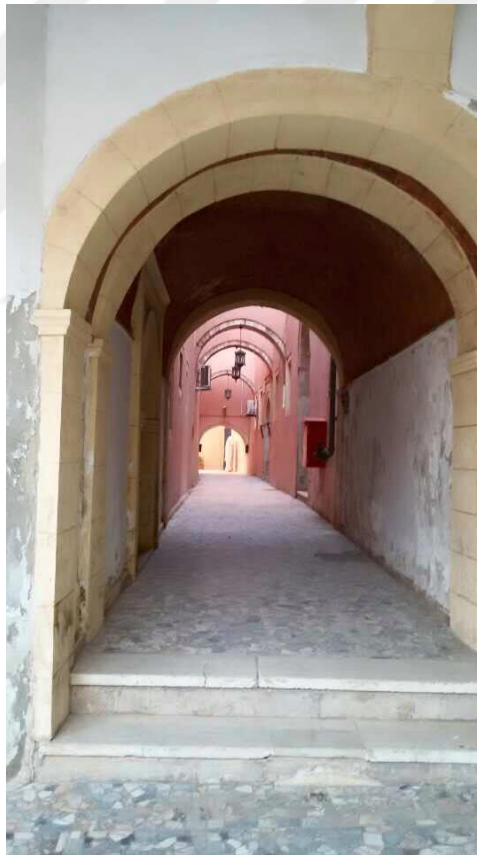
Figure 4.3: Parts of the Red Saraya that received rehabilitation measures and requires minimal repair and intervention. (Author's collection)
