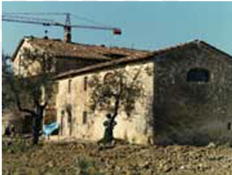
Figure 3.5: Villa Le Torri before restoration (Le Torri, 2013)
