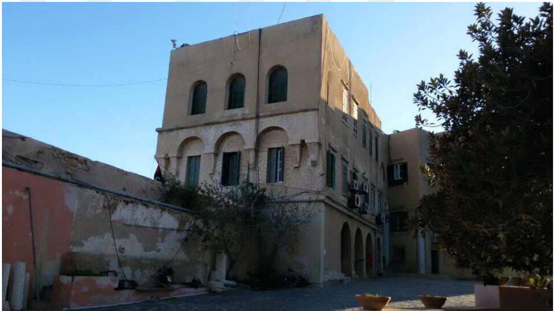
Figure 2.13: A building built during the second Ottoman period (Author's collection)
