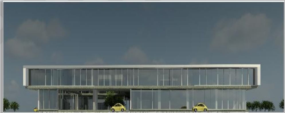
Figure.3.5: Existing building is represented by render program, another outside direction.
