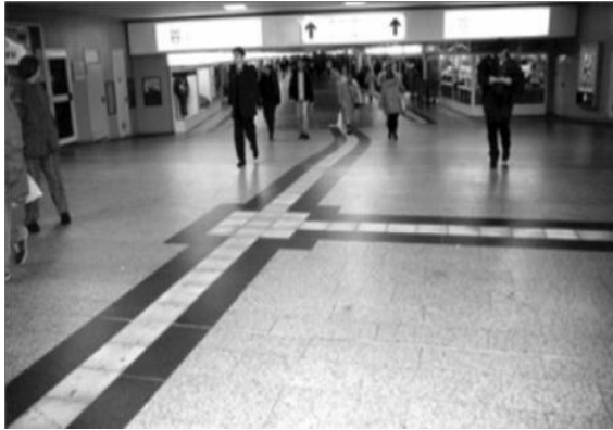
Fig. 3.7. : Example of Guide Tracks (Naniopoulos, 1999)
