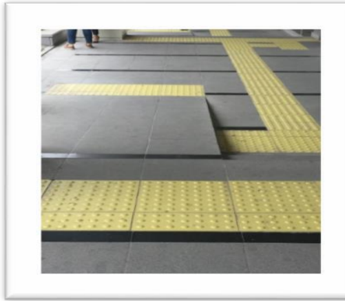
Fig. 4.24. : The Guide Tracks Outside the Building (Self Archive)
