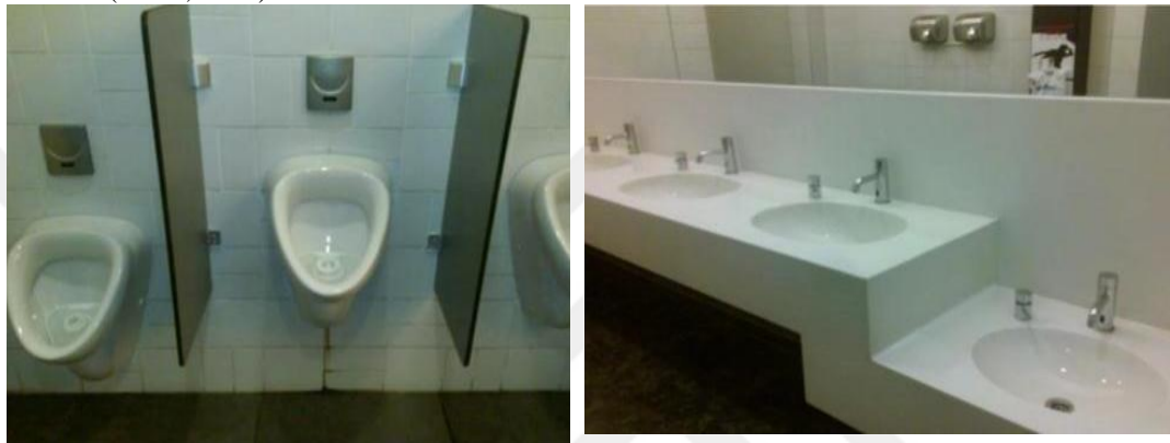
Fig. 4.11. : Urinal and Basin Fixed to Different Heights in Men's Washrooms (Sevük, 2011)
