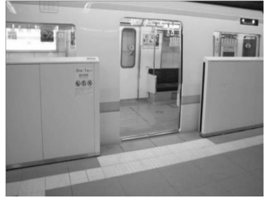
Fig. 3.8. : Orientation of Disabled People with Sensible Surfaces in Urban Rail Stations like Metro (Naniopoulos, 1999)
