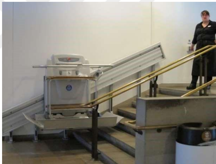
Figure 2.21: Stair lift at Aalto University to increase vertical accessibility (Raike, Ahlava, Akytta, & Tuomi, 2016)
