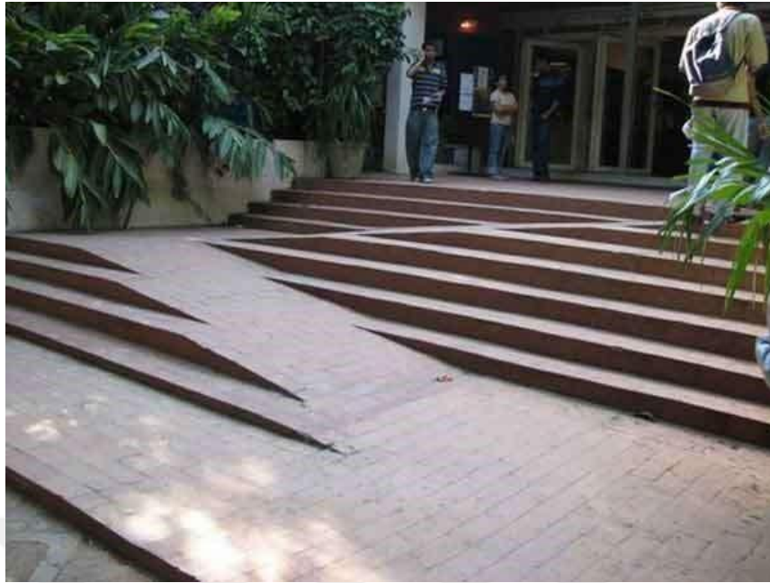
Figure 2.5: Options for usage method illustrated by providing an access using stairs and ramp (Stairs for the Wheels, 2018)
