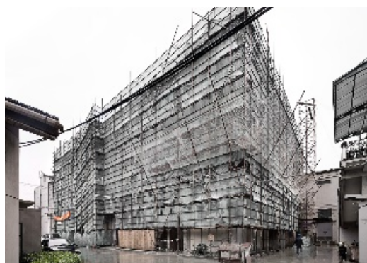
Figure 4.27: Construction View of the Main Building during Transformation of the Glass-Making Factory into SHMOG (Url 4.37)
