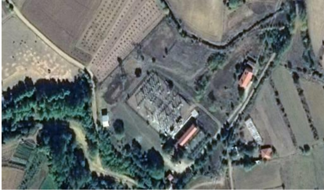
Figure 43 Top view of Taşköprü Substation
