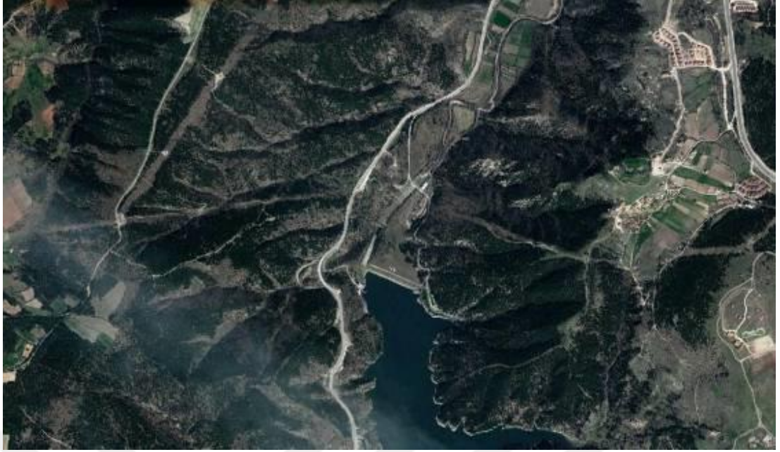
Figure 69 Top view of Karaçomak Dam and its lake in Kastamonu province
