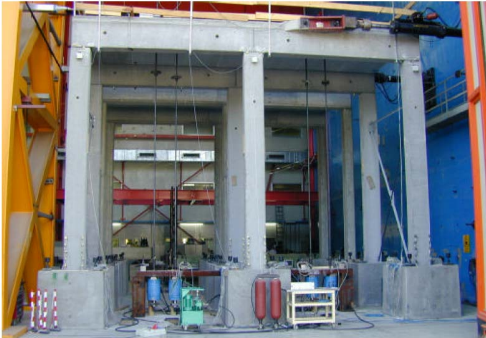
Figure 4.2. The picture of the precast building, Ferrera and Negro (2004)
