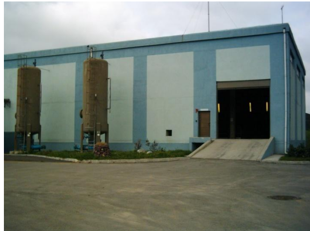
Figure 3.4. Pumping Station of Paşaköy WWTP
