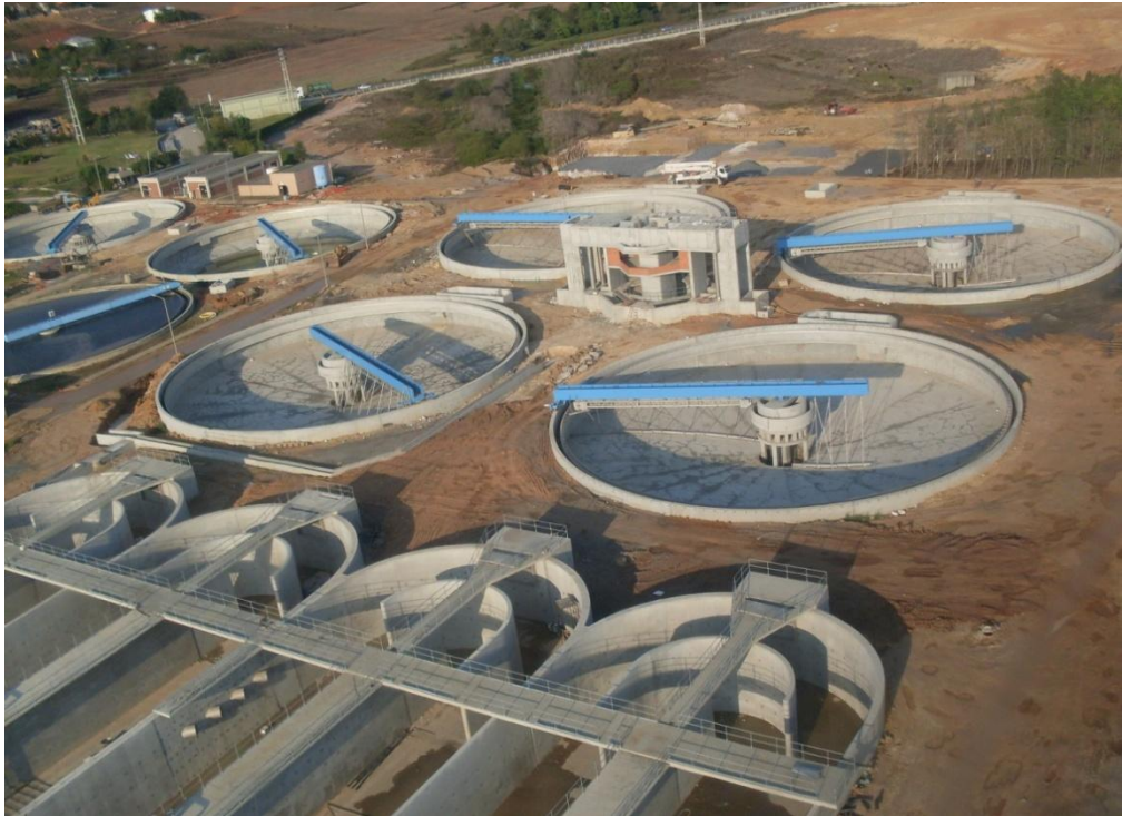
Figure 3.12. Final Clarifiers at Construction State
