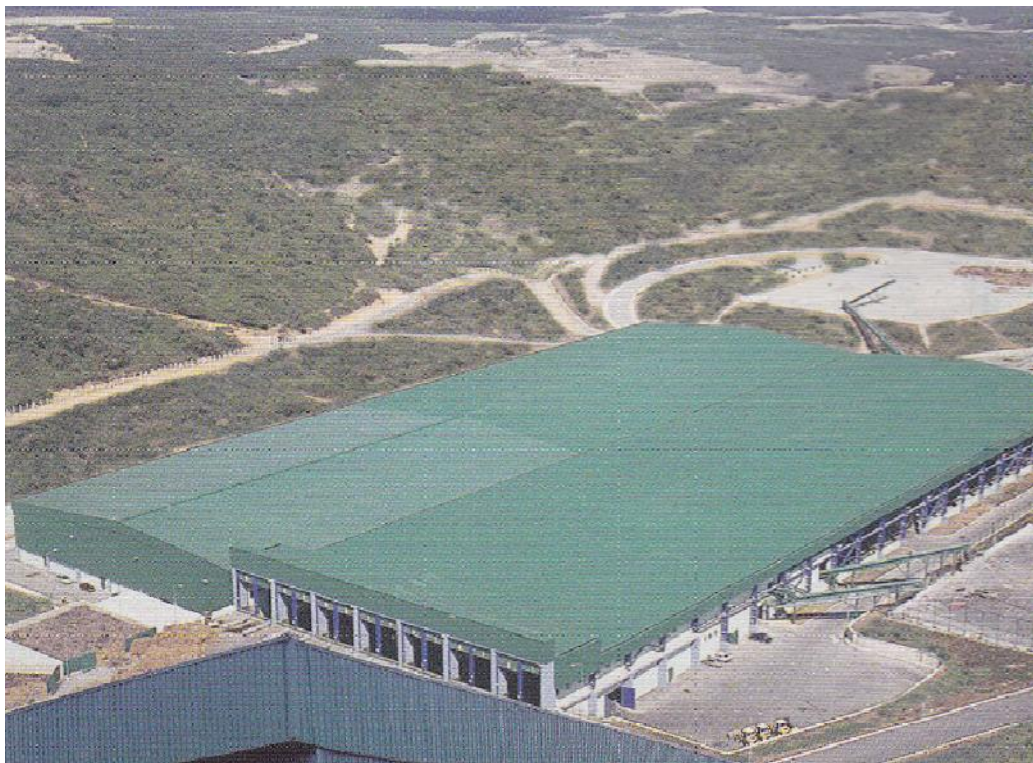
Figure 7.13. Kemberburgaz Compost Facility (İSTAÇ, 2010)
