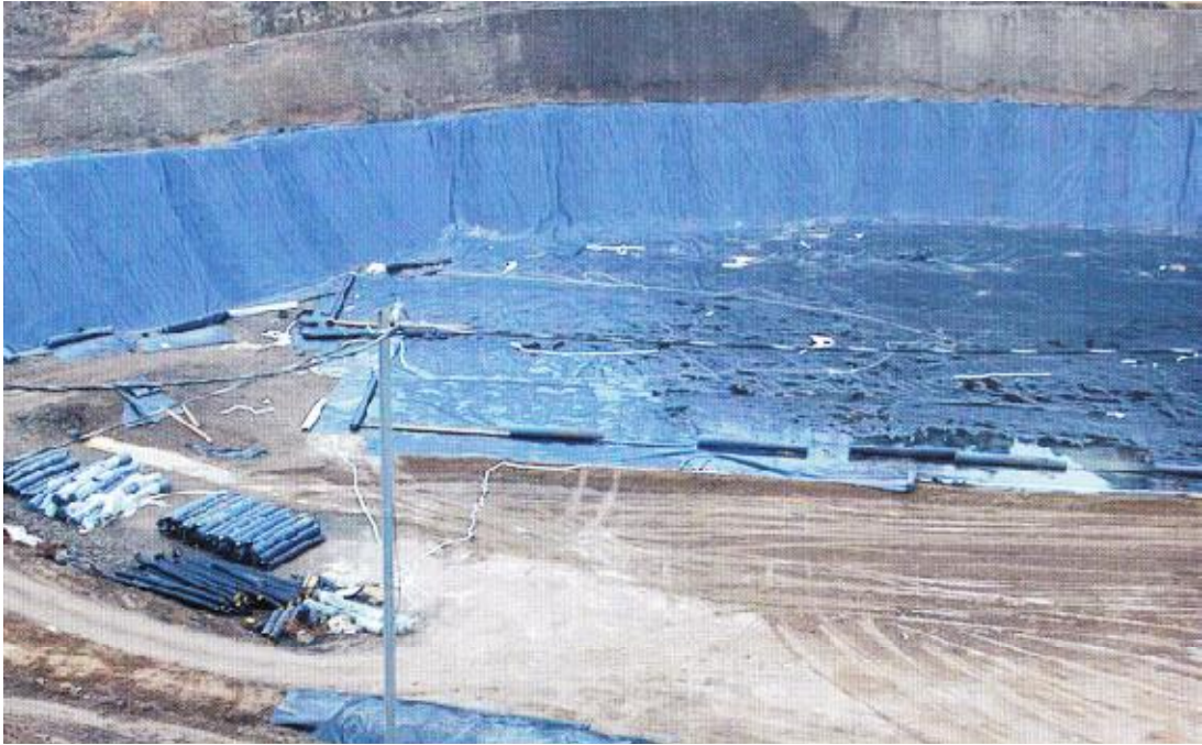
Figure 7.5. Impermeable geomembrane spread under landfill (İSTAÇ, 2010)
