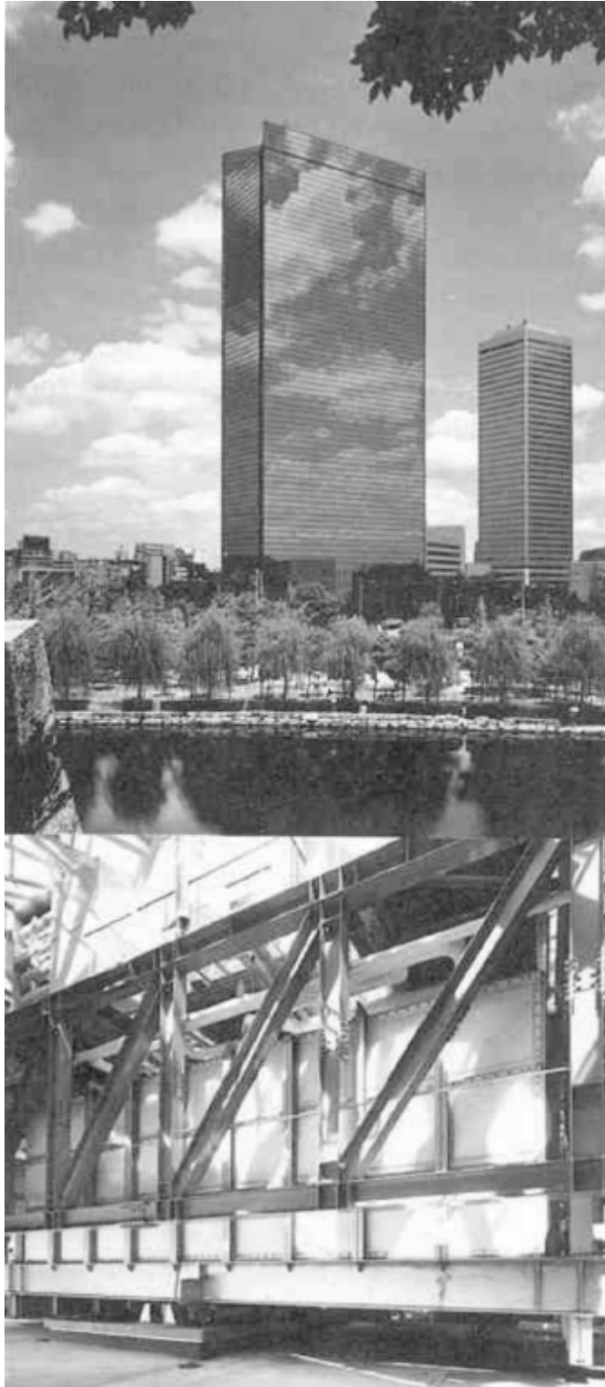
Figure 3.21. Ice storage tank—Crystal Tower. [4]
