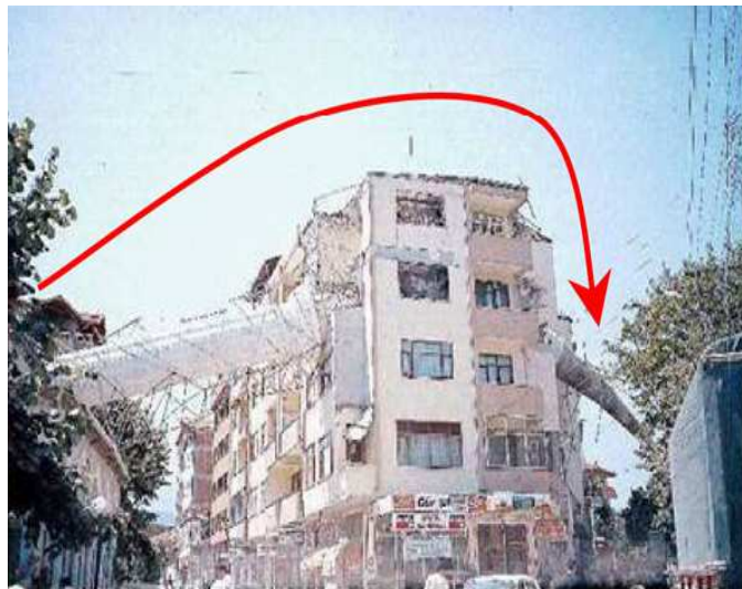
Figure 5.2. Collapse of a minaret onto a nearby building. [5]
