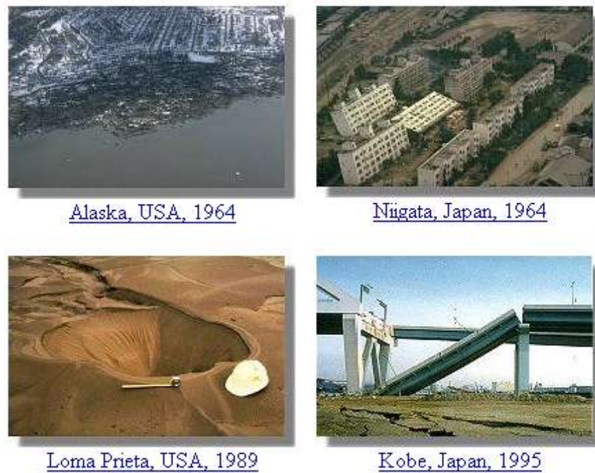
Figure 4.1. Earthquake hazards caused by liquefaction.
