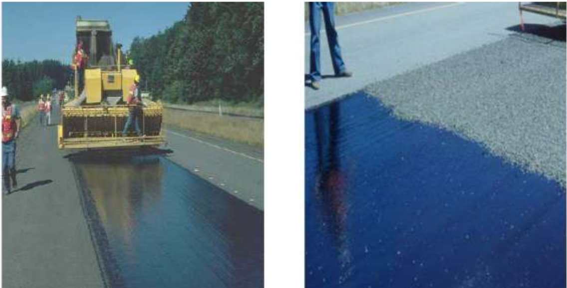
Figure 2.10. Tire chip-seal construction
