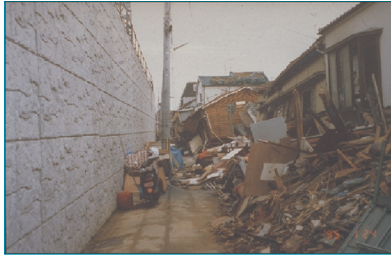
Figure 2.17. Tanata Wall and the around structures after Kobe Earthquake.
