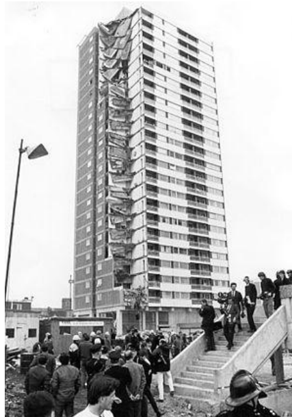
Figure 1.1. Progressive collapse of Ronan Point building (Nair, 2004).
