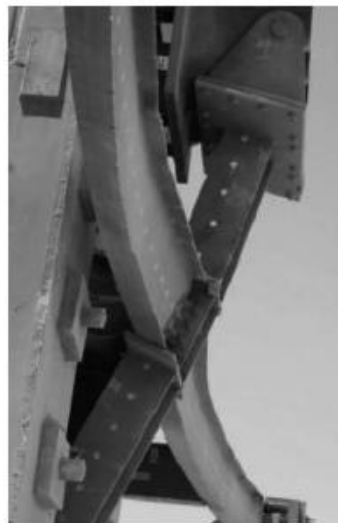
Figure 3.9. Push-down test of damaged steel specimen (Stevens et al. , 2011).
