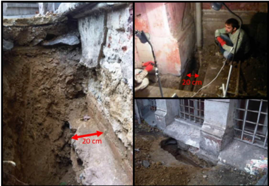
Figure 3.5. Excavation work to determine the foundation system.
