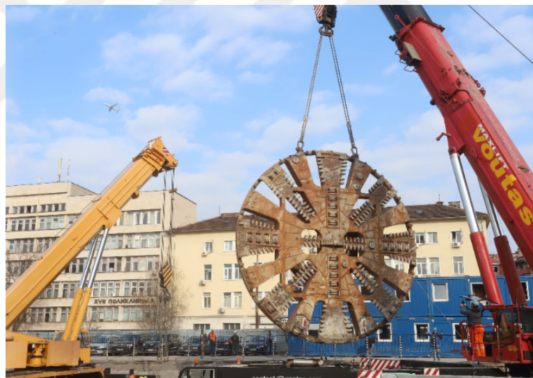
Figure 5.12. Cutterhead during TBM Disassembly.
