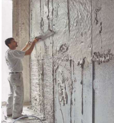
Figure 2.41: PCM plaster applied on interior walls provides thermal insulation, (Leydecker, 2008).
