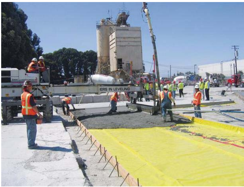
Figure 2.11: An example for fast-drying concrete implementation (Sullivan, 2012).
