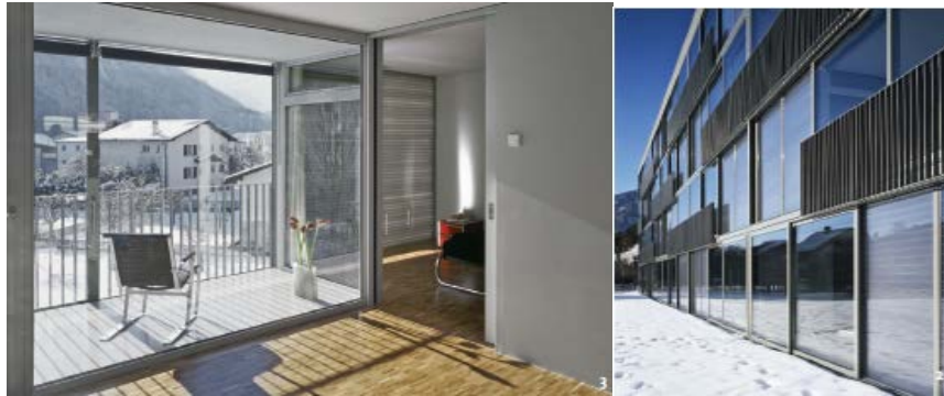
Figure 2.43 and Figure 2.44: Interior and Exterior view of glazed façade with PCM quality, Zurich, Dietrich Schwarz, (Atwa, 2015).
