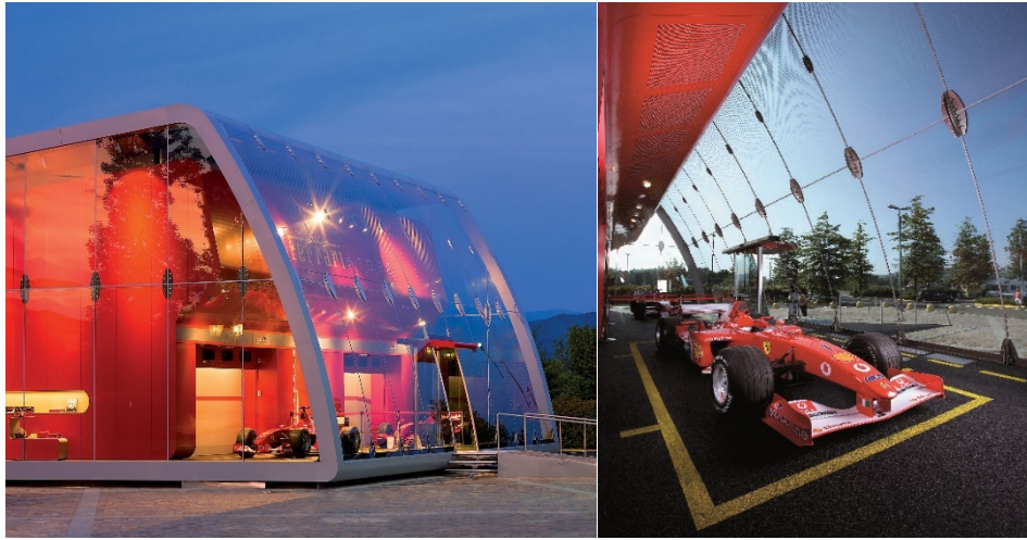
Figure 2.46 and Figure 2.47: outside and inside view of UV protection facade panels of Ferrari Factory Store, Italy, Iosa Ghini Associates, 2009.
