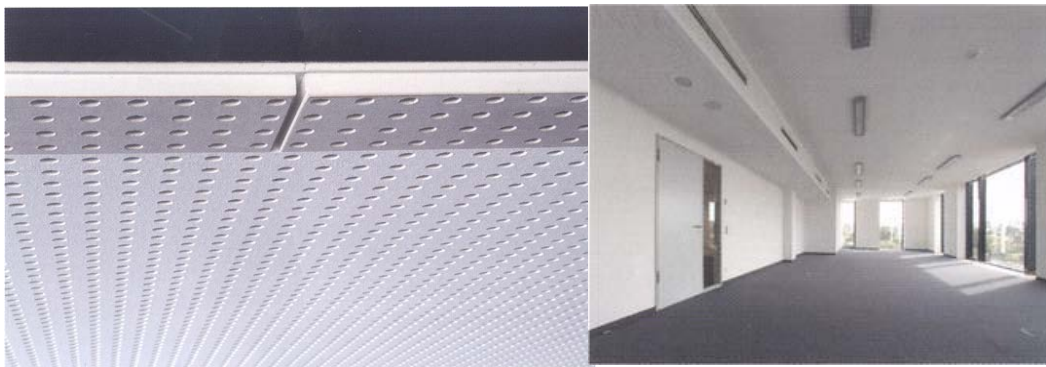
Figure 2.32 and 2.33: Air- purifying materials such as plasterboard oracoustic panels (Leydecker, 2008)
