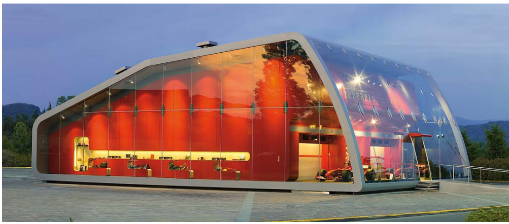
Figure 2.45 UV protecting glasses are used in the facade of Ferrari Factory Store, Italy, Iosa Ghini Associates, 2009.
