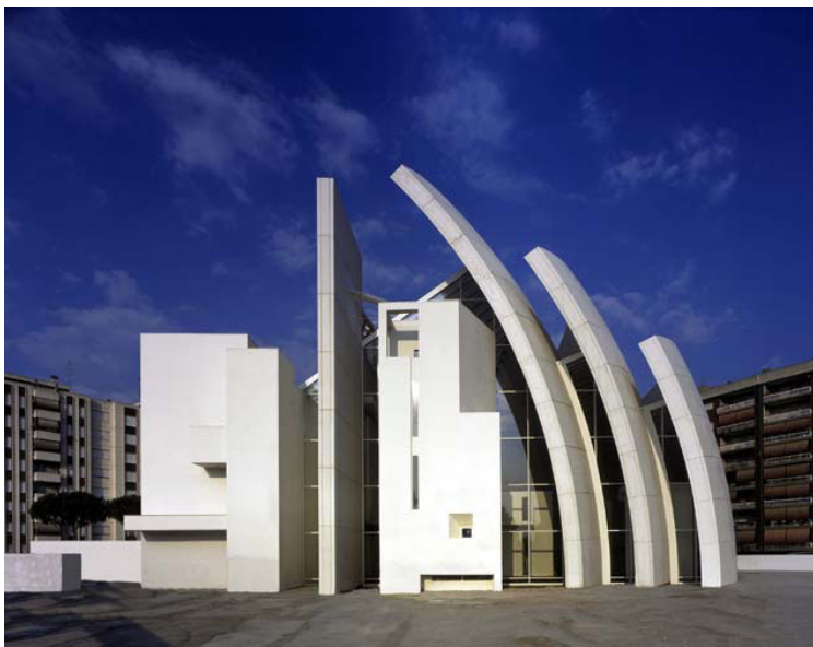
Figure 2.21: White and clean concrete facade of Jubilee church, Rome, Richard Meier, 2003
