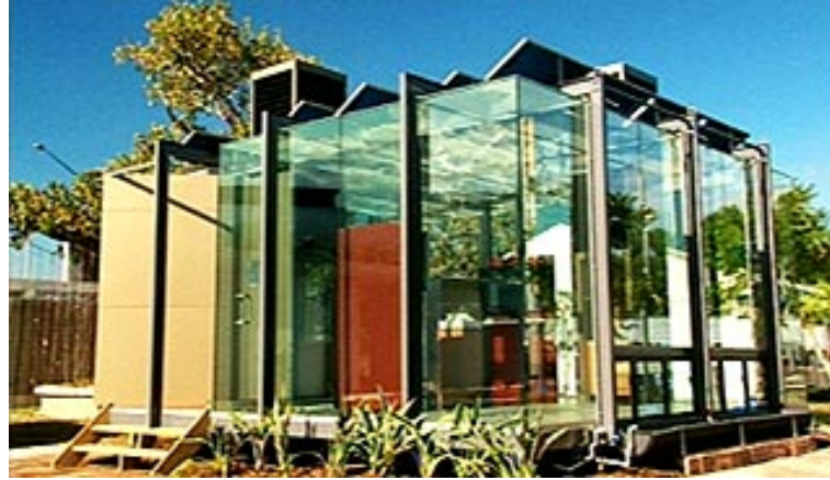
Figure 2.13: The Glass House Project (2004) by architect James Muir, in Nano-house Research Group, CSIRO-Industrial Research Organization and Sydney University of Technology, Dr.Michael Cortie (co), Sydney, 2002.
