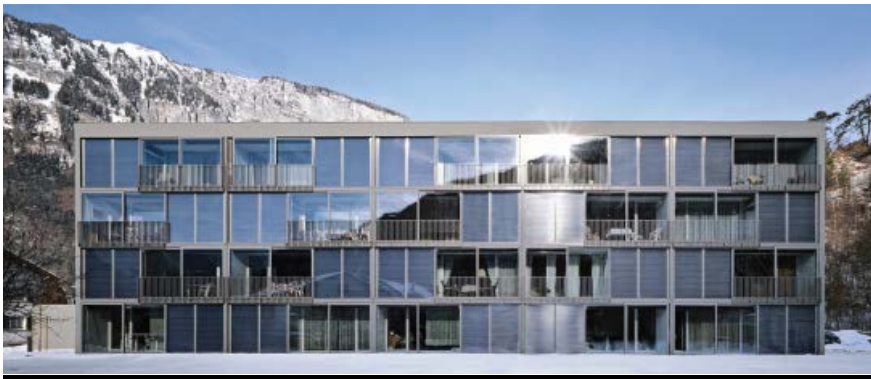
Figure 2.42: Glazed south façade of Sur Falveng with PCM Quality, Zurich, Dietrich Schwarz, (Atwa, 2015).
