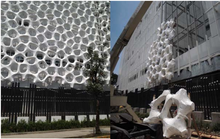
Figure 2.35 and figure 2.36: Prosolve tiles coated with TiO_2 , Mexico City, 2013.
