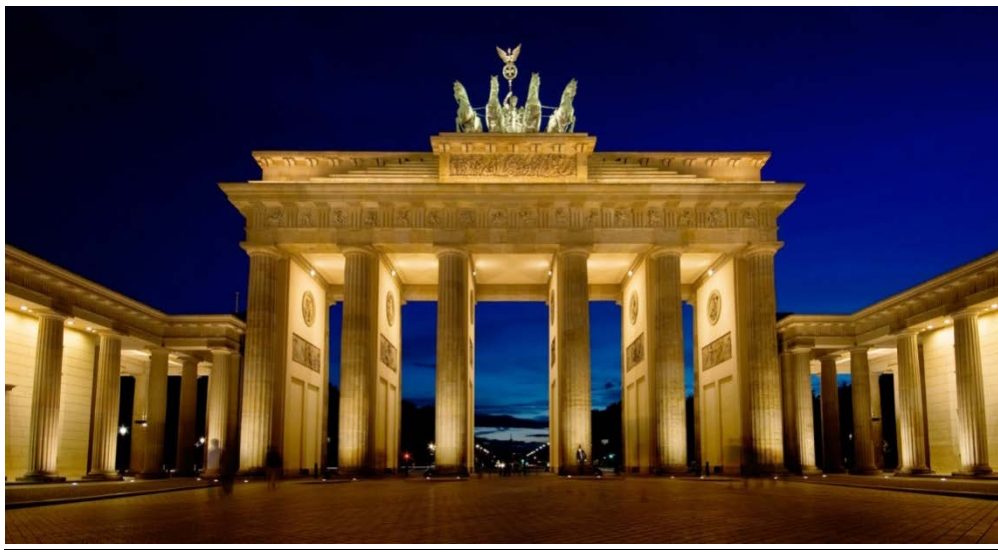
Figure 2.53: Brandenburg Gate, Germany
