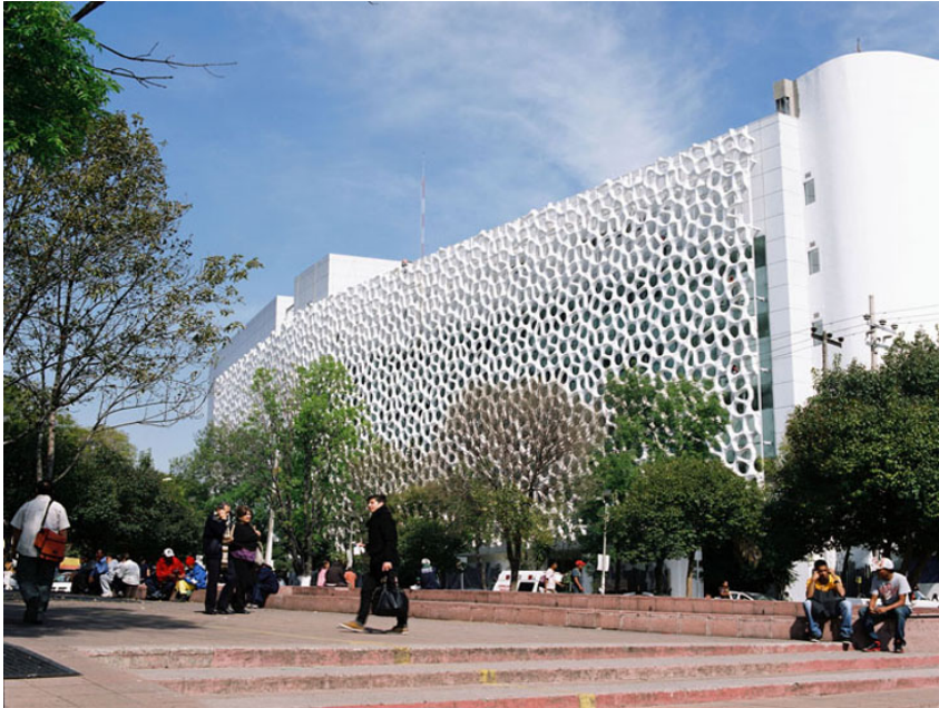
Figure 2.34: Façade of the Manuel Gea González Hospital, Mexico City, 2013.
