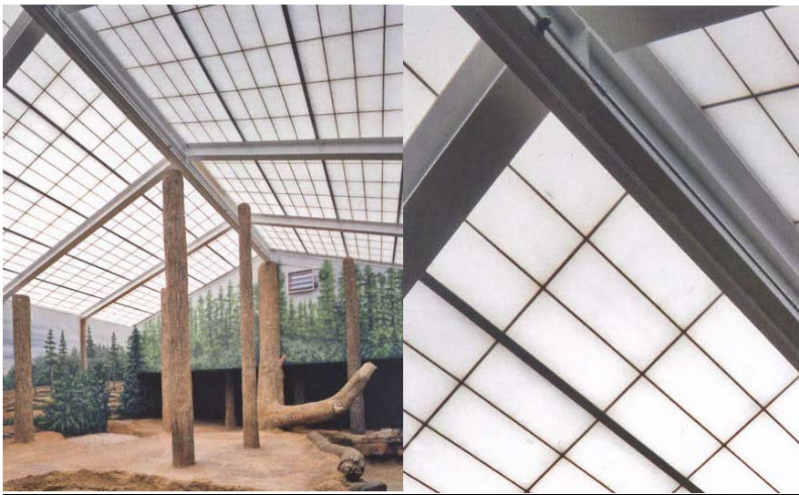
Figure 2.39 and Figure 2.40: Milwaukee County Zoo designed with aerogel-filled glass panels, USA, Zimmerman Design Group, 2005 (Leydecker, 2008).
