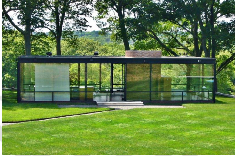
Şekil 25. Glass House, Philip Johnson, 1949
