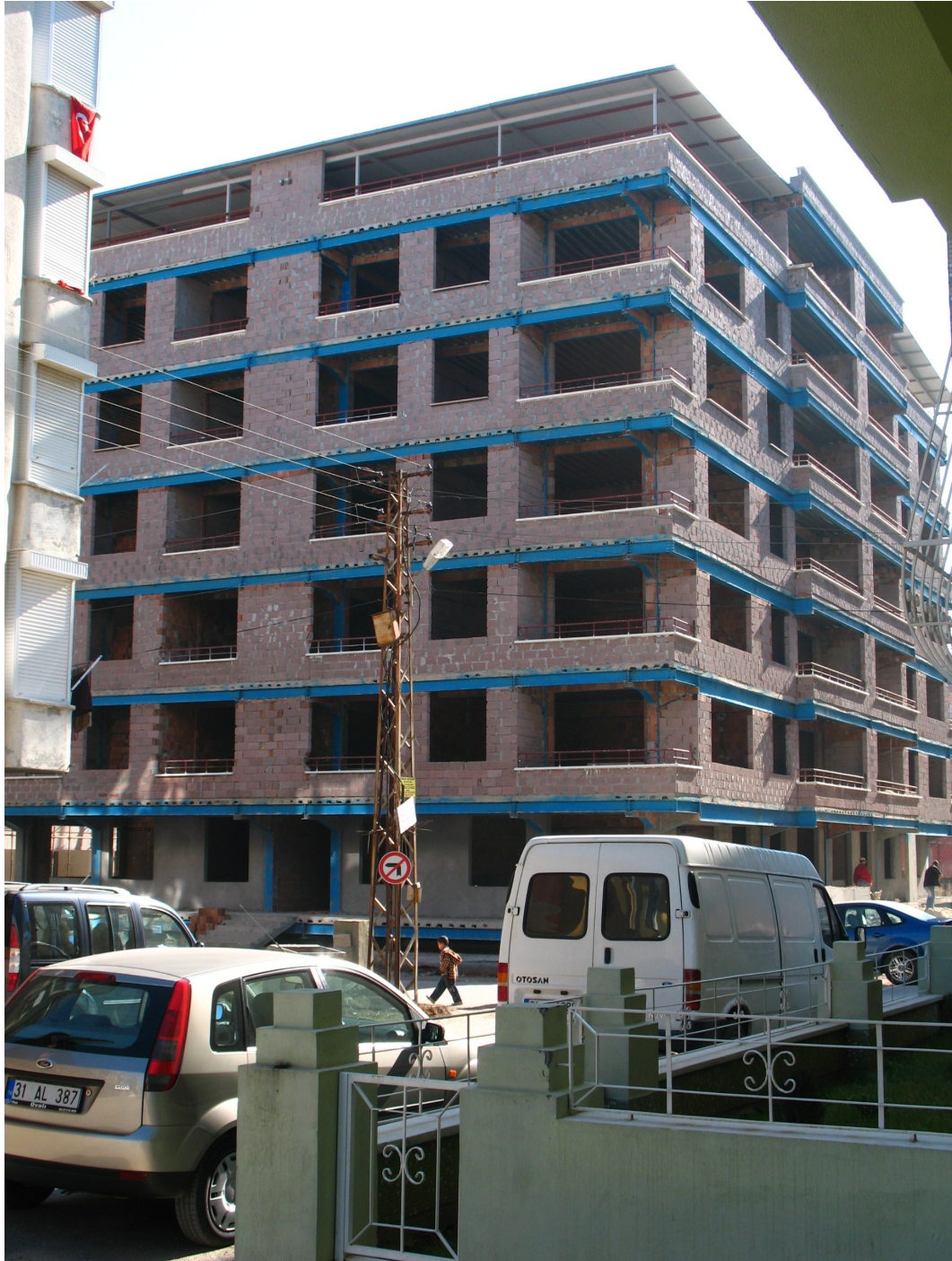
Figure 3.1. Six-story steel hinged-framed building
