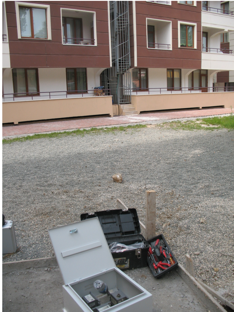
Figure 3.8. Showing the building-free located away from the main building
